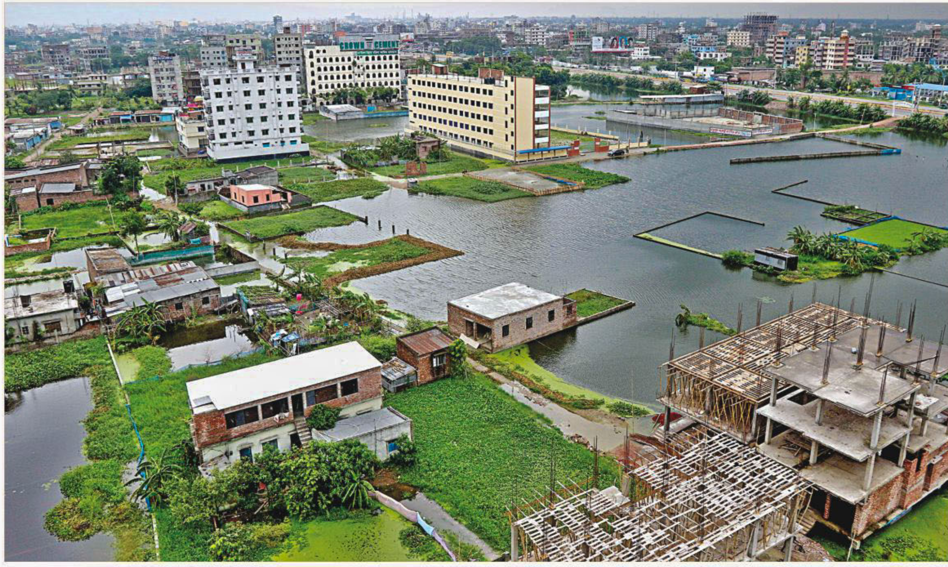
Rain over the last two days has inundated parts of the DND dam area in Matuail of Dhaka. A number of canals, which used to drain the water out, have been blocked up by illegal structures. If rain continues, many more houses in the area may soon be submerged. PHOTO: ANISUR RAHMAN
