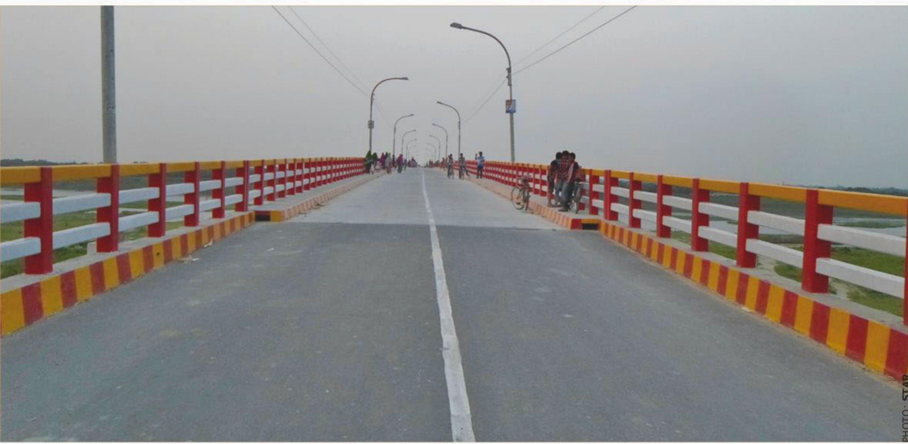
The Sheikh Hasina bridge on the Mohananda River at Shaheber Ghat of Sadar upazila in Chapainawabganj was officially inaugurated on May 16, 2015.
