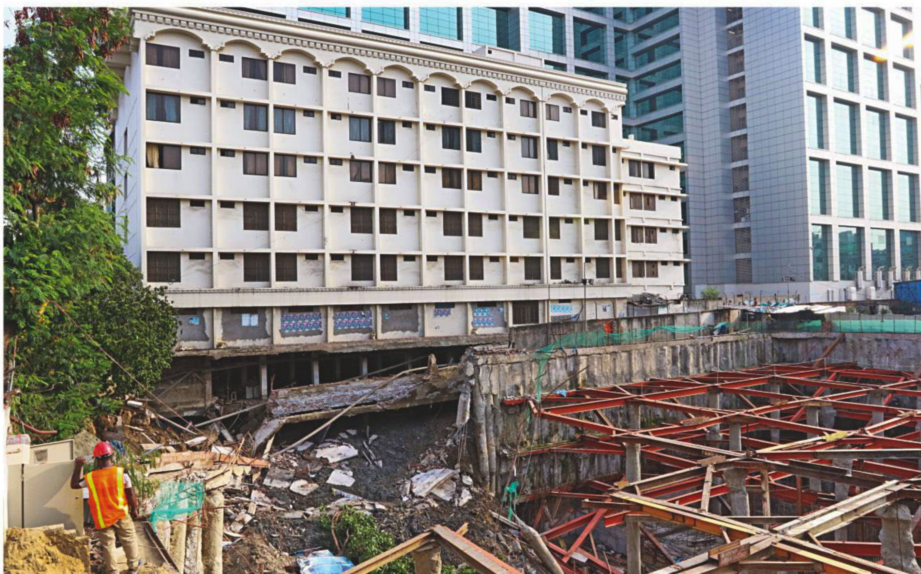
The concrete reinforcement pillars placed for the construction of a new building next to Hotel Sundarban near Sonargaon intersection in the capital gave way yesterday and tonnes of soil from under the hotel slid.
