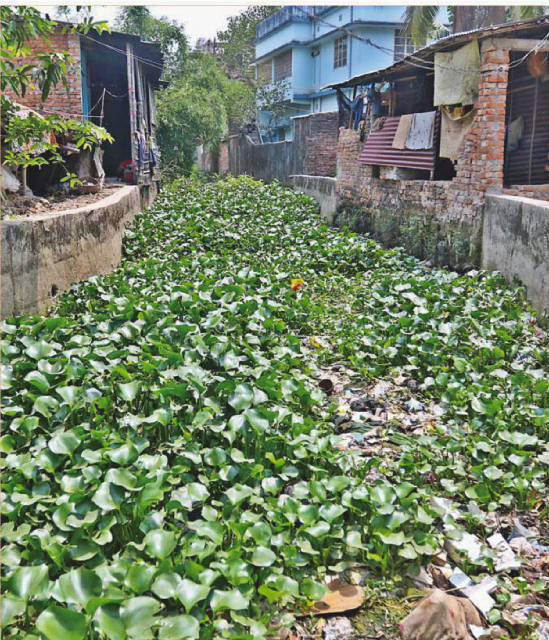
This half kilometre portion of Chaktai Khal is completely covered with water hyacinths in Chittagong city's Bakalia area. The major parts of the canal stretching around 12 kilometres from Bahaddarhat to Karnaphuli river have been narrowed down due to encroachment for a long time. The adjoining areas are waterlogged as the water body cannot carry rain and flood water to the river during the monsoon. Despite repeated assurance from the city corporation authorities, the canal is yet to be saved from grabbing and pollution. The photo was taken recently.
