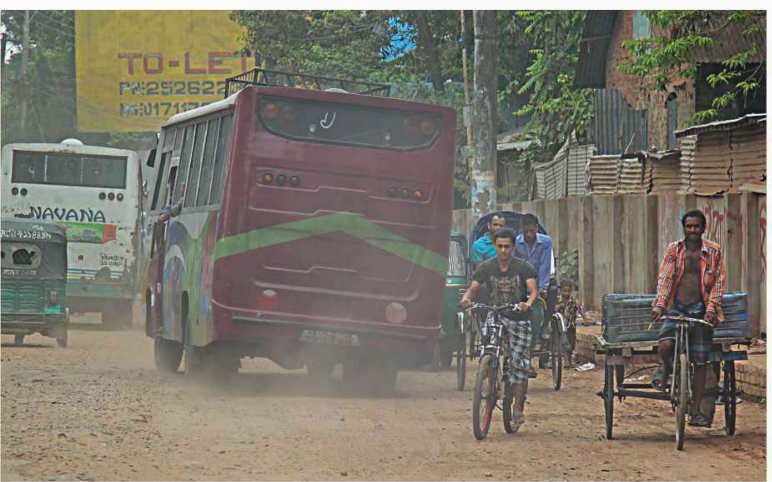
Dust hampers the movement of people between BRTC area and Kadamtali of Chittagong city where a 1.1km flyover is under construction. The work is supposed to be completed in June but may get extended till September. The photo was taken at Kadamtali intersection yesterday.
