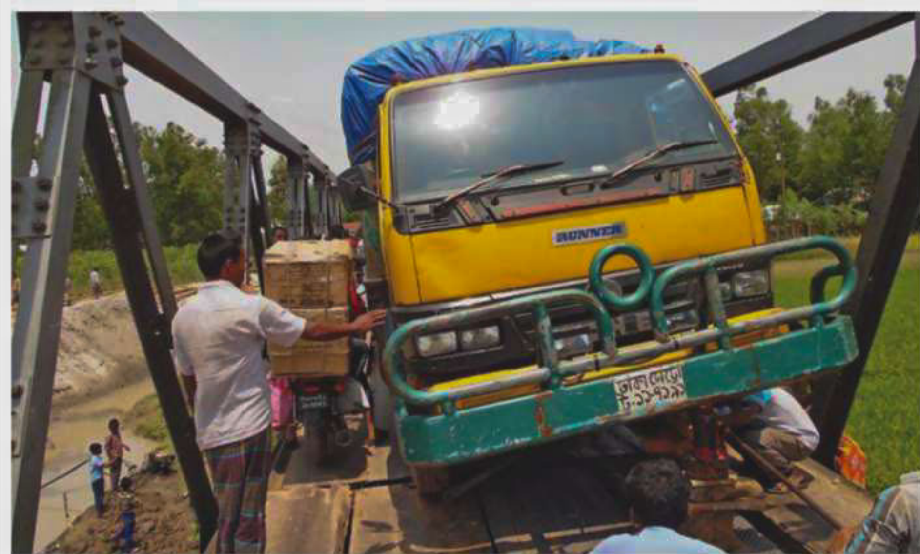
A heavily loaded truck got stuck on this Bailey bridge over the Jamuneshwari River at Hortukitola village in Nilphamari Sadar upazila after its wheels slipped into the gap of displaced steel plates on the deck on Monday, snapping direct vehicular movement on Nilphamari-Panchagarh road. The bridge remains highly vulnerable as activists of Jamaat-e-Islami and its student wing Islami Chhatra Shibir caused serious damage to the structure during their violent political agitation on December 12 in 2013 but the Roads and Highways Department did only a few temporary repairs since then.
