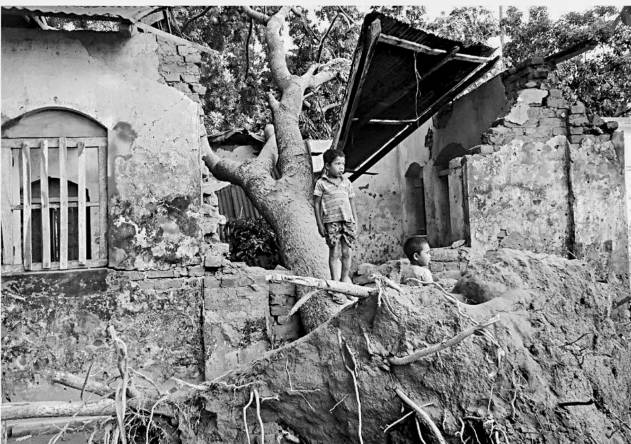
The building of Osmania High School in Trishal upazila under Mymensingh district lies ravaged as a nor'wester lashed the area on Saturday night.
