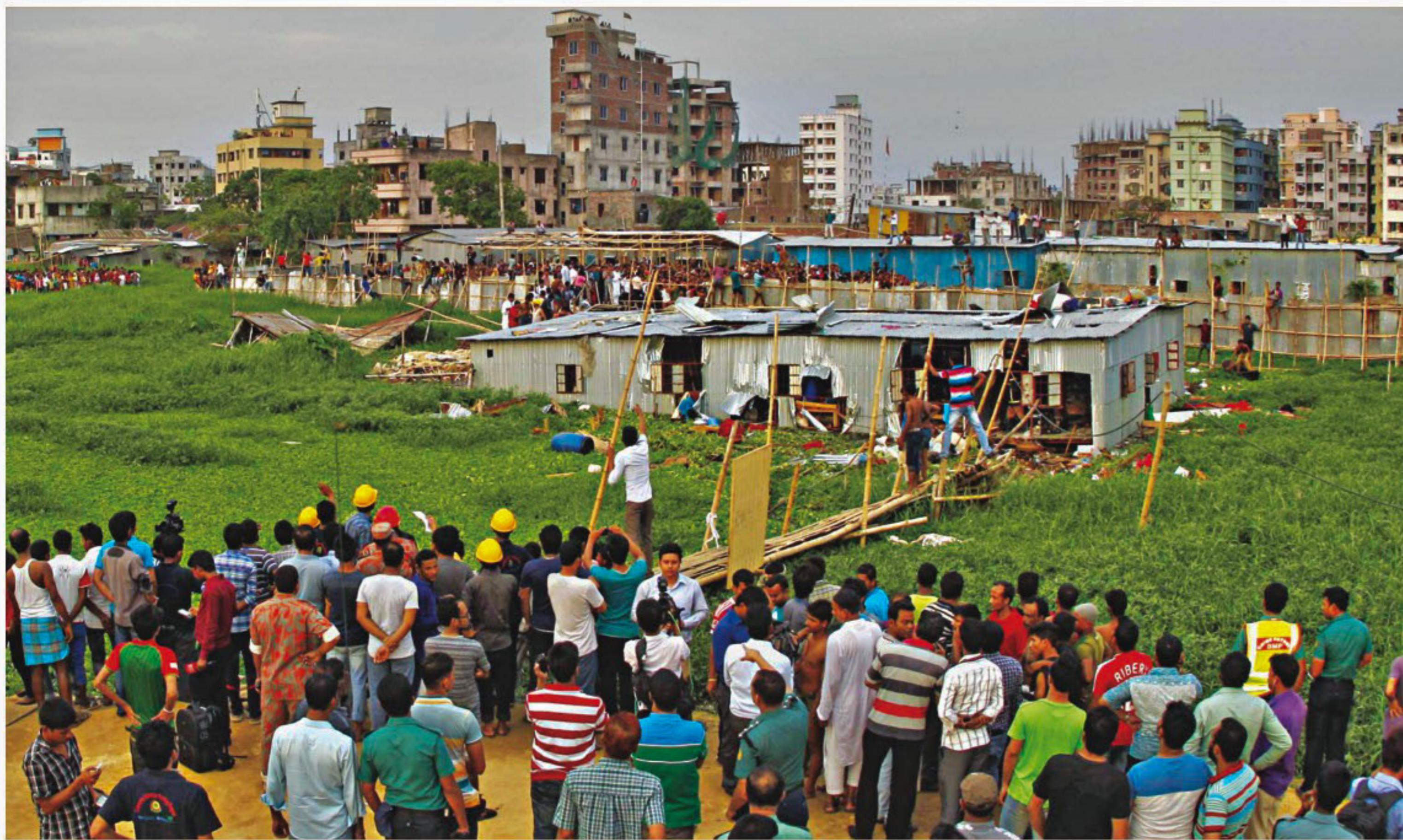
Onlookers and rescuers gather at a marshland in the capital's Rampura yesterday after a large two-storey structure made of corrugated iron sheets over the water went down. Only the first floor of the structure is visible and the "ground floor" has gone under water. The house had 20 rooms in which an estimated 120 people lived.
