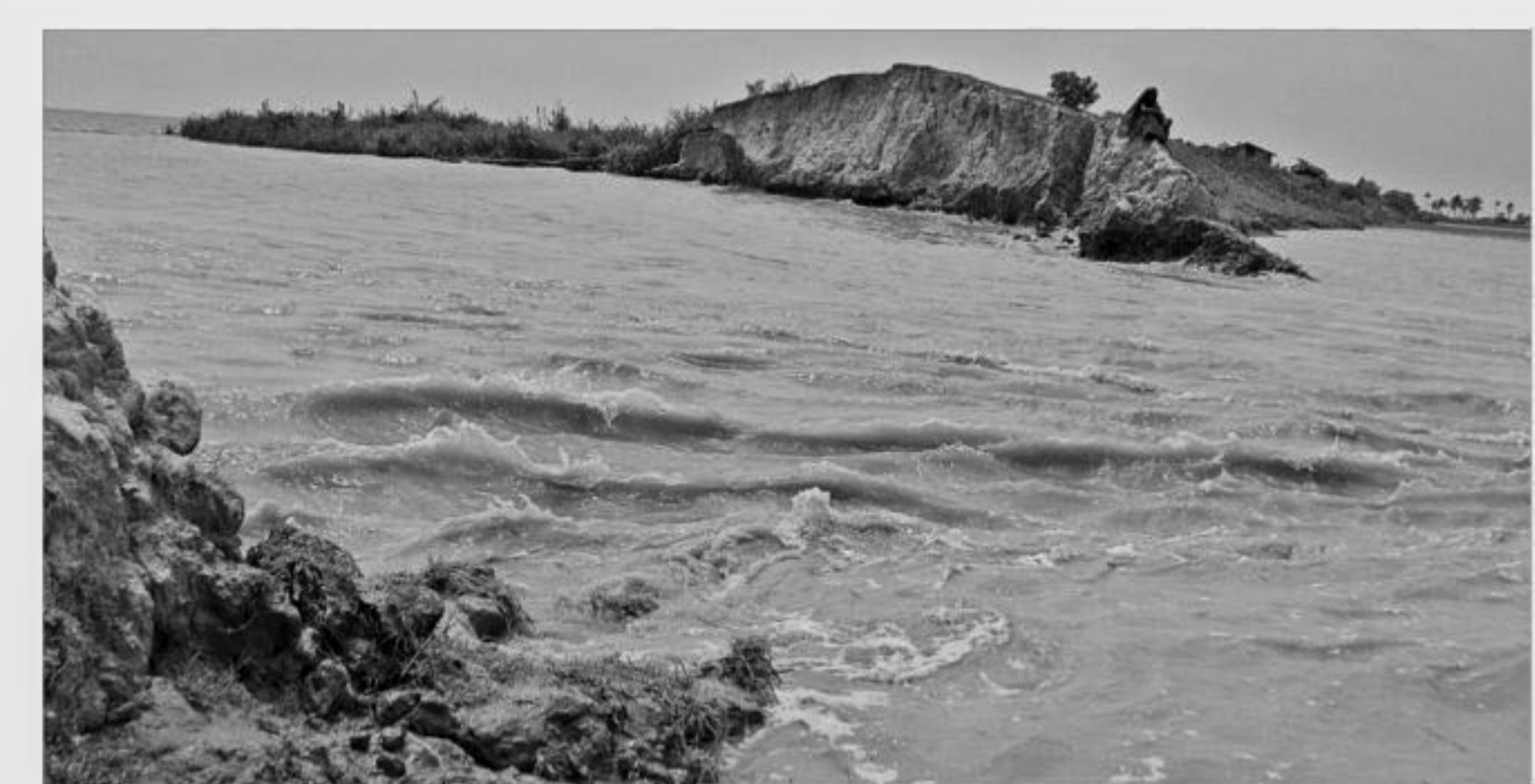
The swelling Ramnabadh River at Lalua union of Patuakhali inundated five villages yesterday as the embankment there has not been repaired yet after being breached last year. PHOTO: ARIFUR RAHMAN
