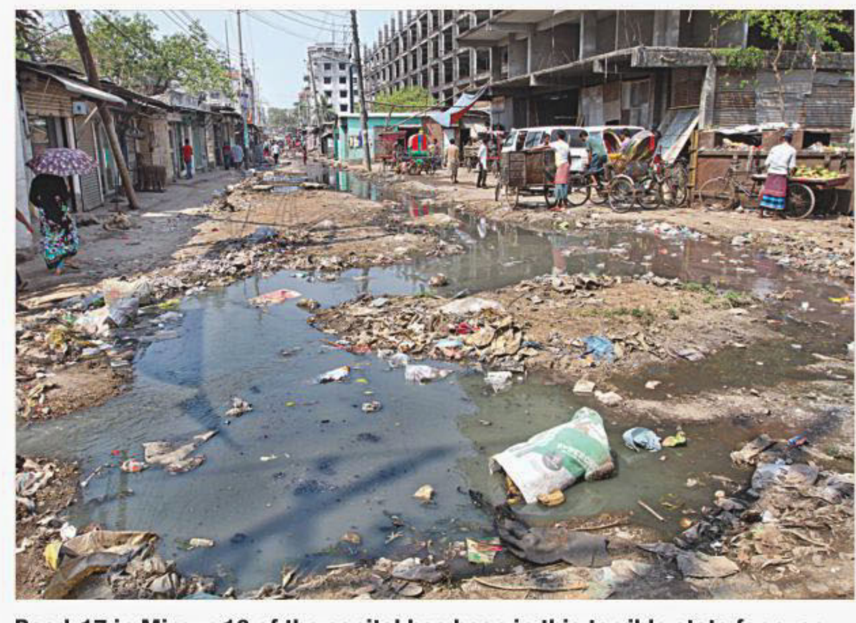
Road-17 in Mirpur-10 of the capital has been in this terrible state for over three years. The road is usually, if not always, flooded with sewage causing misery to pedestrians and residents. The photo was taken recently.
