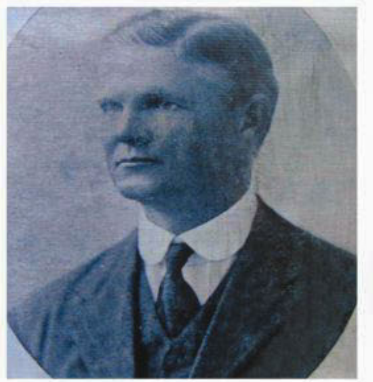
Mr. Gayle, Engineer in charge of construction of Hardinge Bridge
