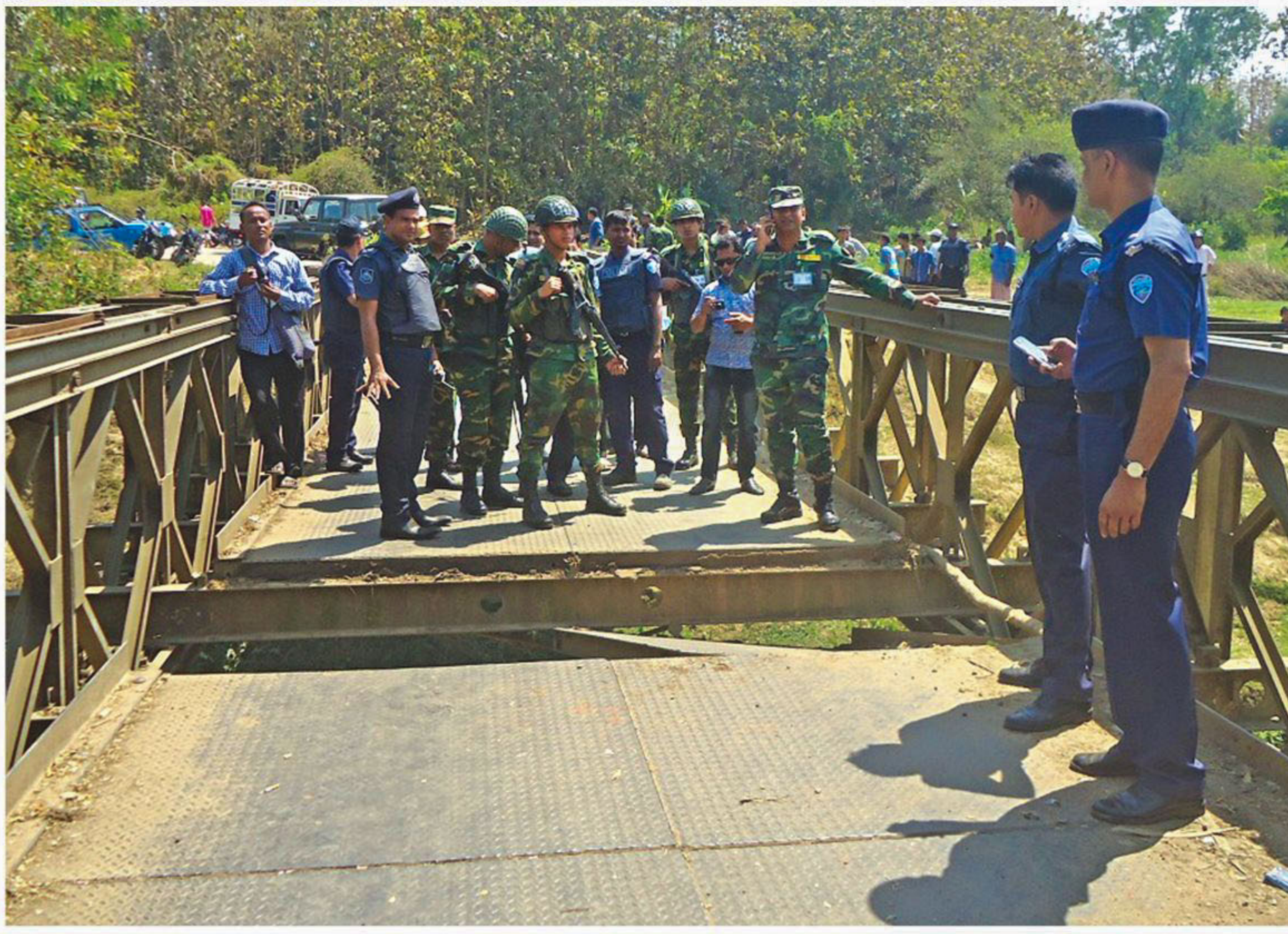
Law enforcers and armed forces personnel inspect a Bailey bridge on Bandarban-Rangamati road in Sonar Mandir area yesterday. Criminals took two plates of the bridge off, disrupting vehicular movement on the road for around an hour.
