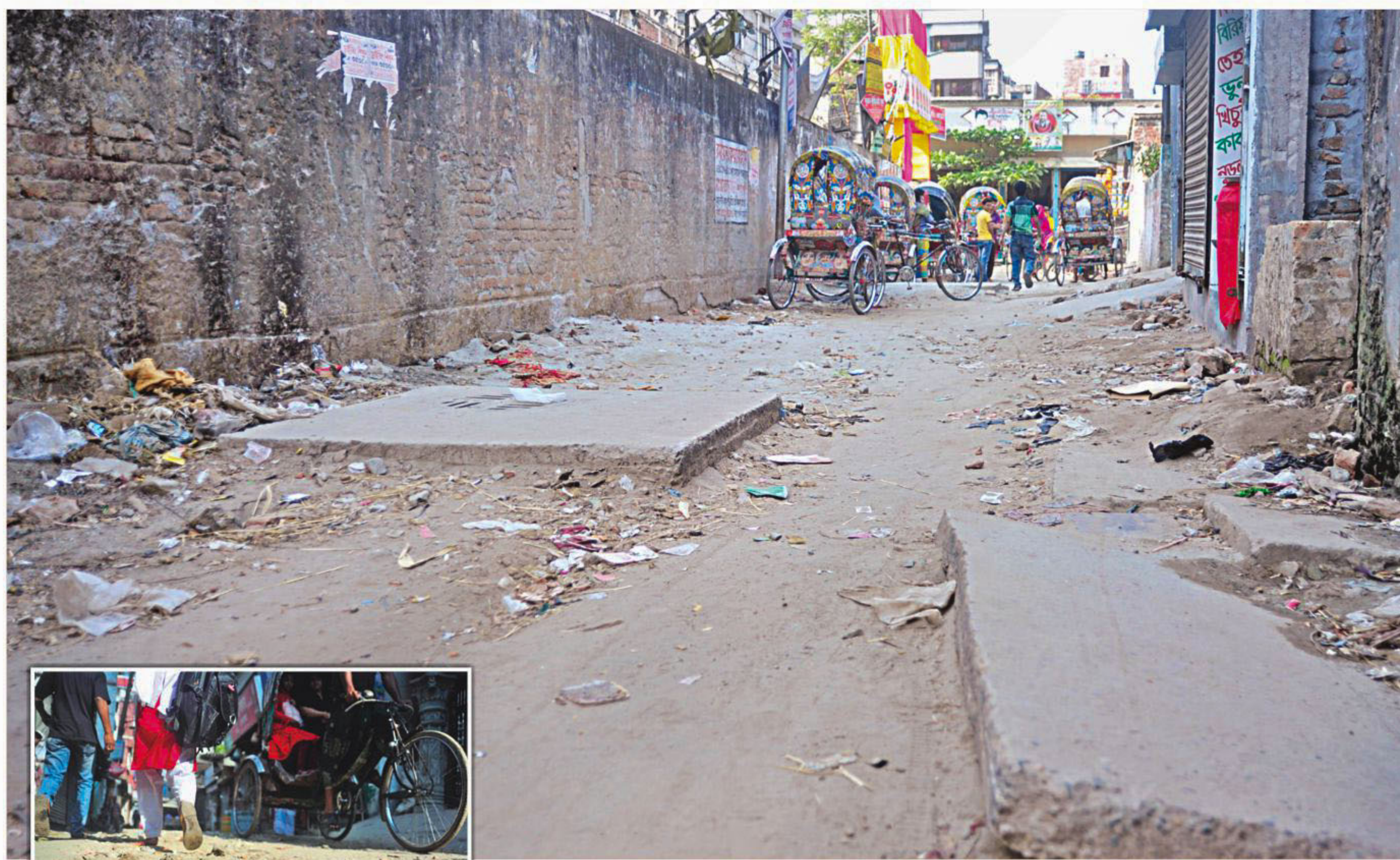
Concrete manhole covers protruding on the surface make it extremely difficult for vehicles to ply an already dilapidated Chandan Kotha Road in Jatrabari. Inset, stones and pieces of bricks on the road as Dhaka South City Corporation did not repair it after placing a sewerage line underneath the road six months back. The photo was taken yesterday.
