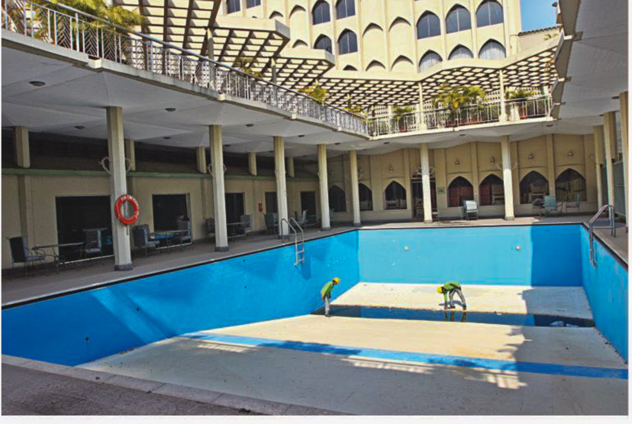
Two men work at the swimming pool of Ruposhi Bangla as part of the renovations of the hotel.
