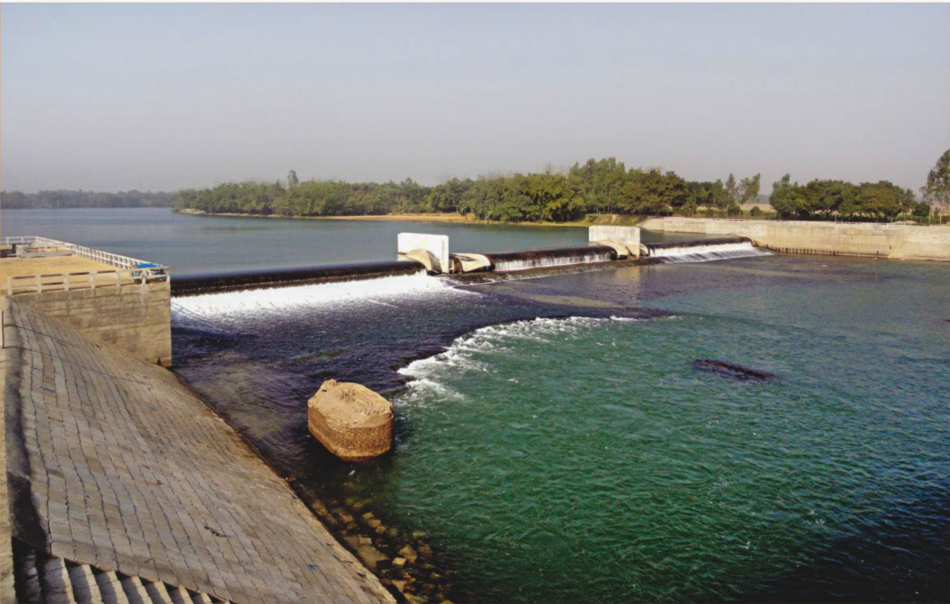
The newly constructed rubber dam on the Atrai in Mohonpur of Dinajpur has been raising the water level of the river since the middle of this month so that farmers have easier access to irrigation water during the dry season.
