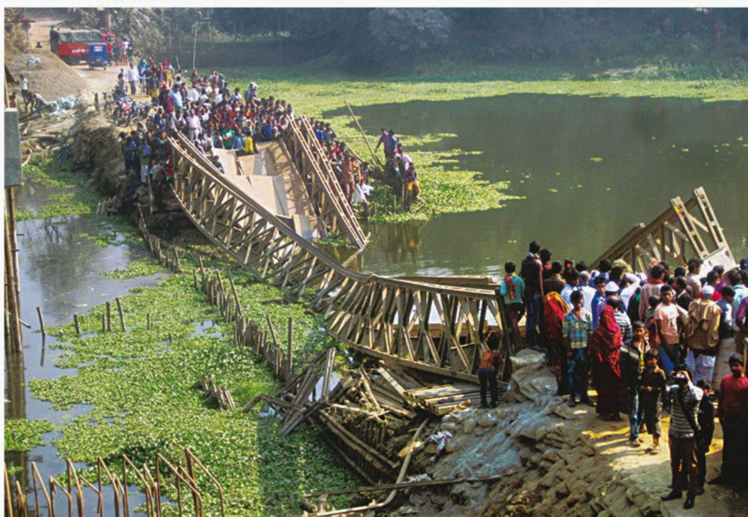
The wreckage of a bailey bridge at Kiting Char in Manikganj's Singair upazila. It collapsed after a stone-laden truck tried to cross the already-dilapidated bridge, killing the driver and his assistant. Road communication between the upazila and Dhaka was snapped following the incident.
