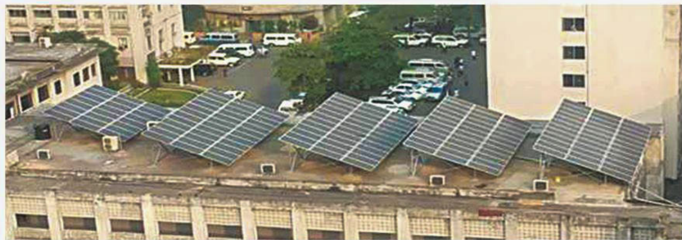
With no batteries in the system, this solar power plant on the Secretariat supplies 50kw electricity to the national grid.
