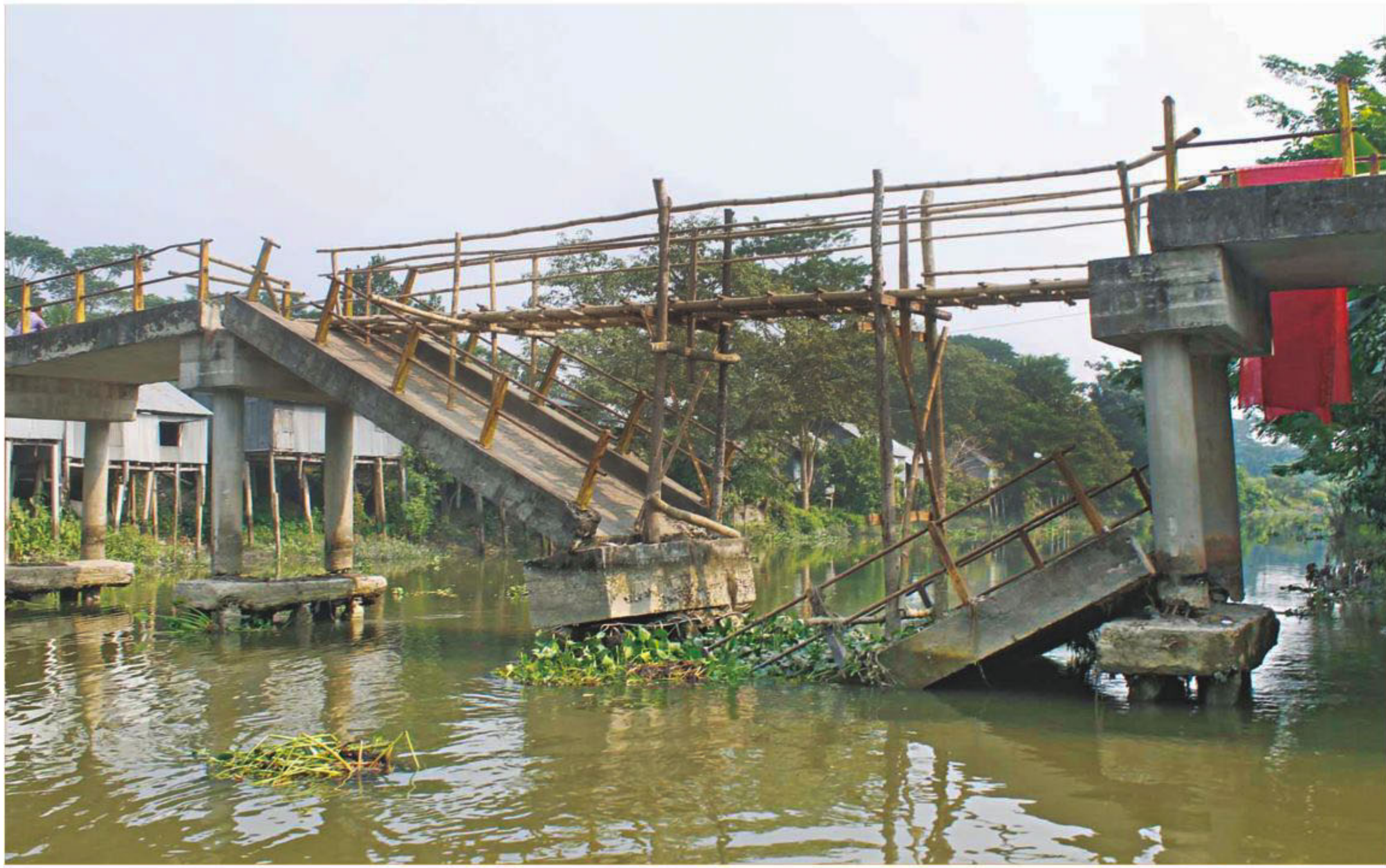
The bridge on the road between Bakal and Bagdha unions of Agailjhara upazila in Barisal has been like this for over two years. Locals have built a bamboo structure over the broken part so that people could cross. The authorities seem to have no intention to repair it.
