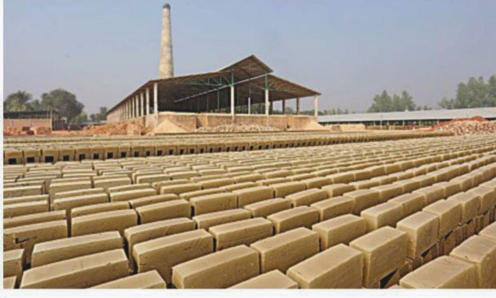
PHOTO: STAR The coalyard at Barapukuria Coalmine in Dinajpur remains empty as production was suspended in May for a sudden surge of water in the underground. Although the authorities resumed mining in November, they were yet to restart supply to the brickfields 'for raising coal stock'. Inset, a brickfield sits idle and counts losses for want of coal in its peak season in Bogra.
