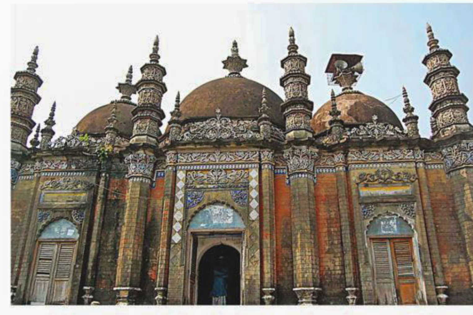
The photos of historic Karapur Mian Bari Mosque at Uttar Karapur in Barisal Sadar before and after renovation easily show the differences in their colours.
