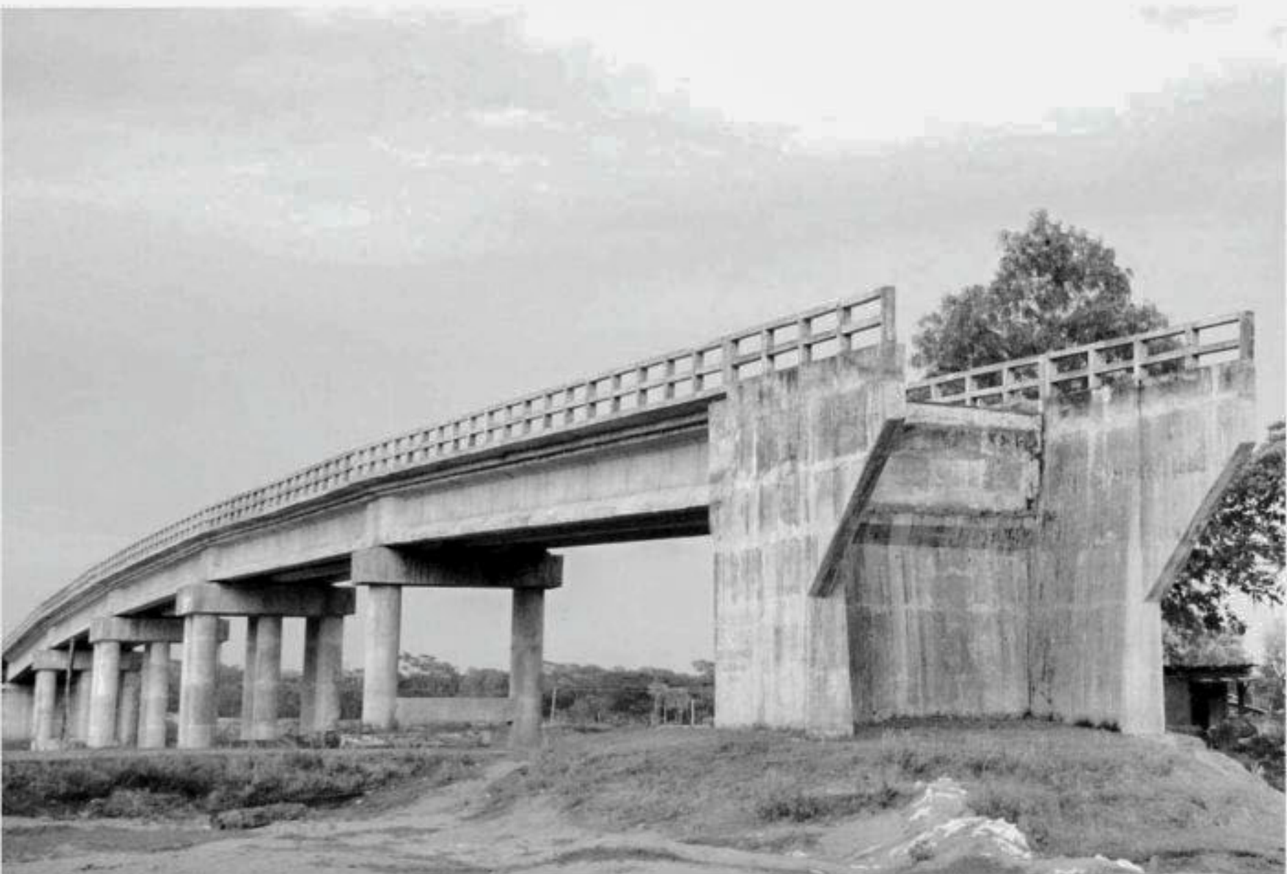
The bridge on Nurainpur canal in Baufal upazila under Patuakhali district, and right, another one on Kalishuri canal in the same upazila, have remained unusable as the authorities concerned did not bother to build approach roads, respectively six and two years after completion of the bridges.
