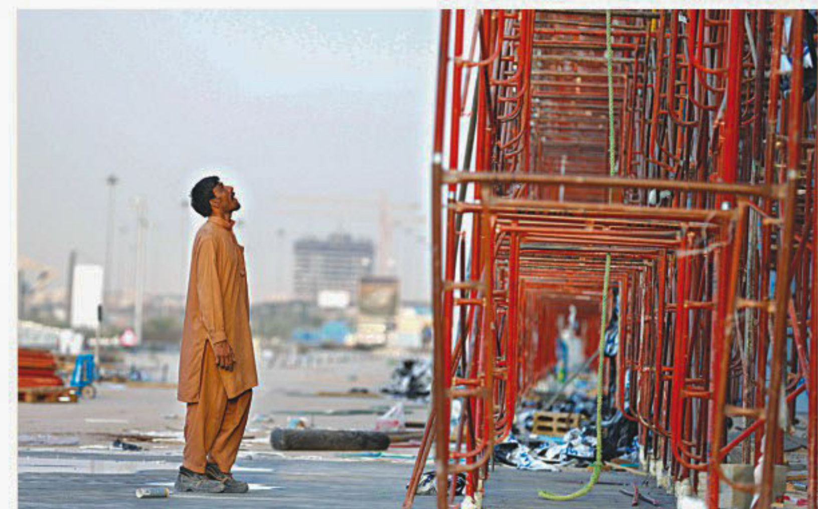
An Indian labourer looks at the construction site of a building in Riyadh.
