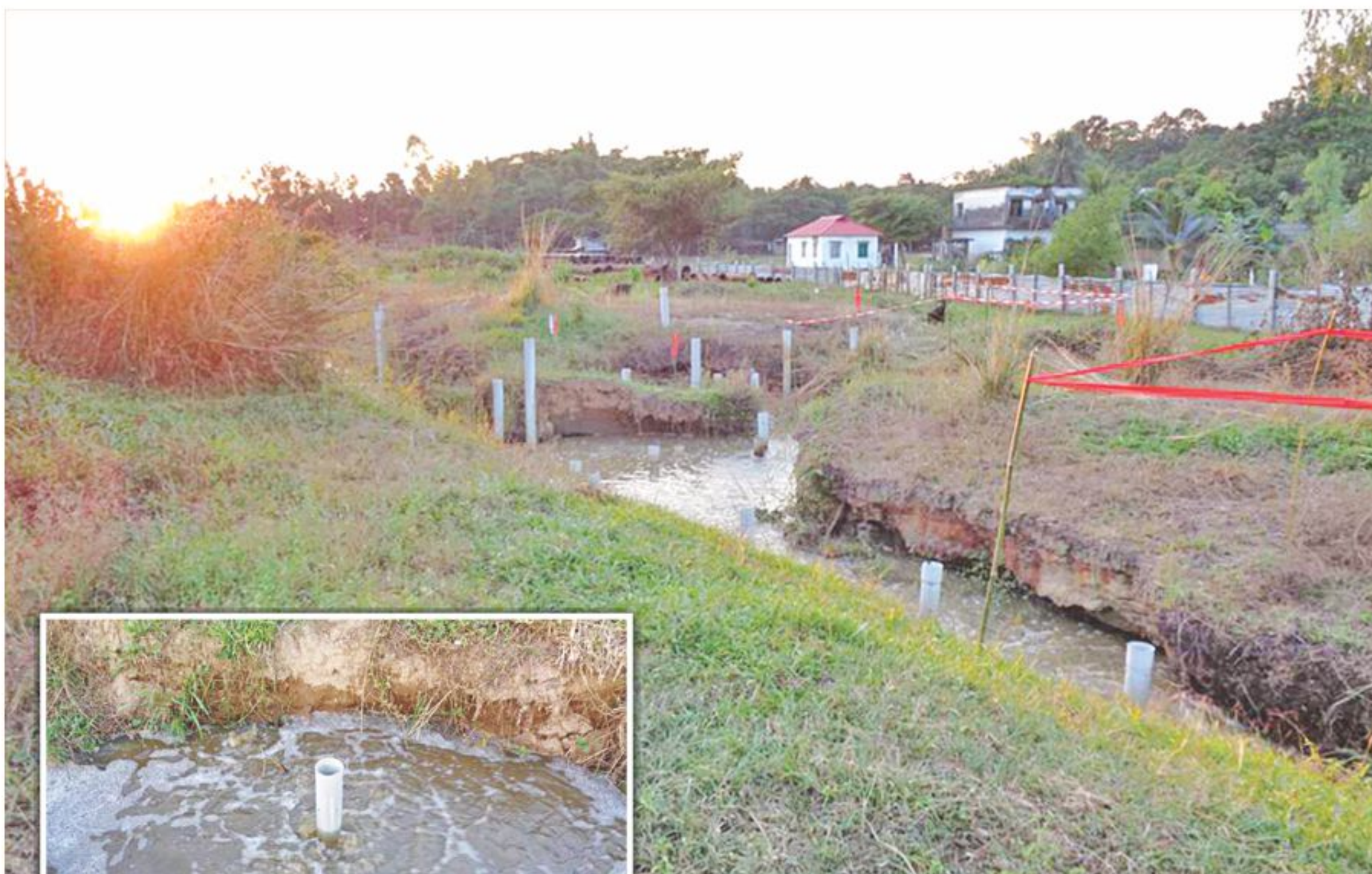
Pipes set in Tengratila gas field in Sunamganj to ease a sudden intensification of leakage, inset, coming to notice a couple of days ago. The gas field had been abandoned since two big blowouts occurred during well drilling in 2005. The photos were taken yesterday.
