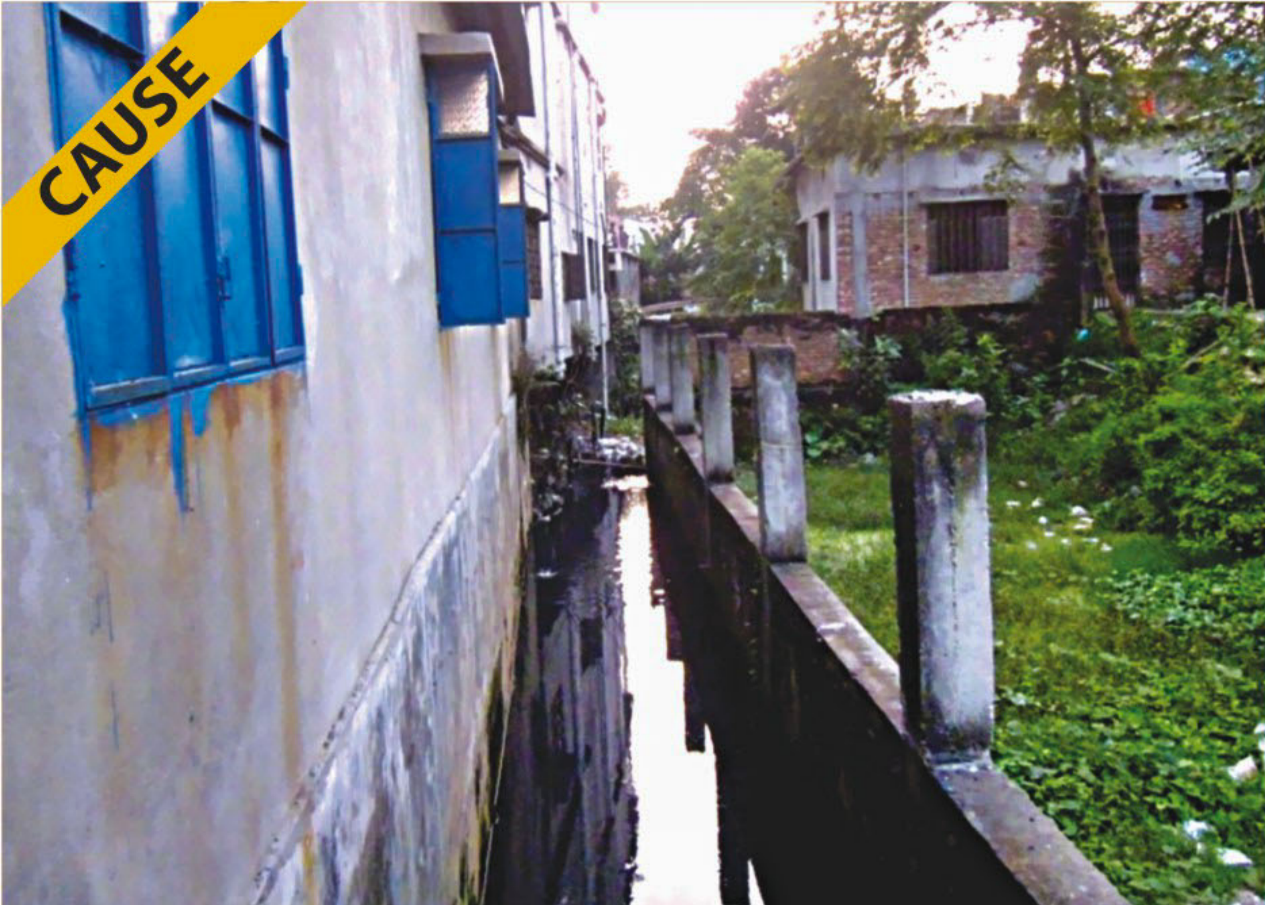
This building and the adjacent structures, left, have been built smack in the middle of what used to be Boiragirbari Khal in Savar on the outskirts of the capital, encroaching upon the canal, which used to be 60 to 80 feet wide, stretching for 2.5 kilometres, carrying rain and flood water to the Dhaleshwari river during the monsoon. Now because of the encroachment even a moderate rainfall creates a 4 to 5 feet deep waterlogging in Bank Colony and Talbagh areas, right next to Dhaka-Aricha highway, right. The encroachment has been going on for the last 20 years by the local influential quarters, building multi-storey structures in and around it. The authorities concerned claimed that the encroachers keep coming back despite their eviction drives. The photos were taken recently.
