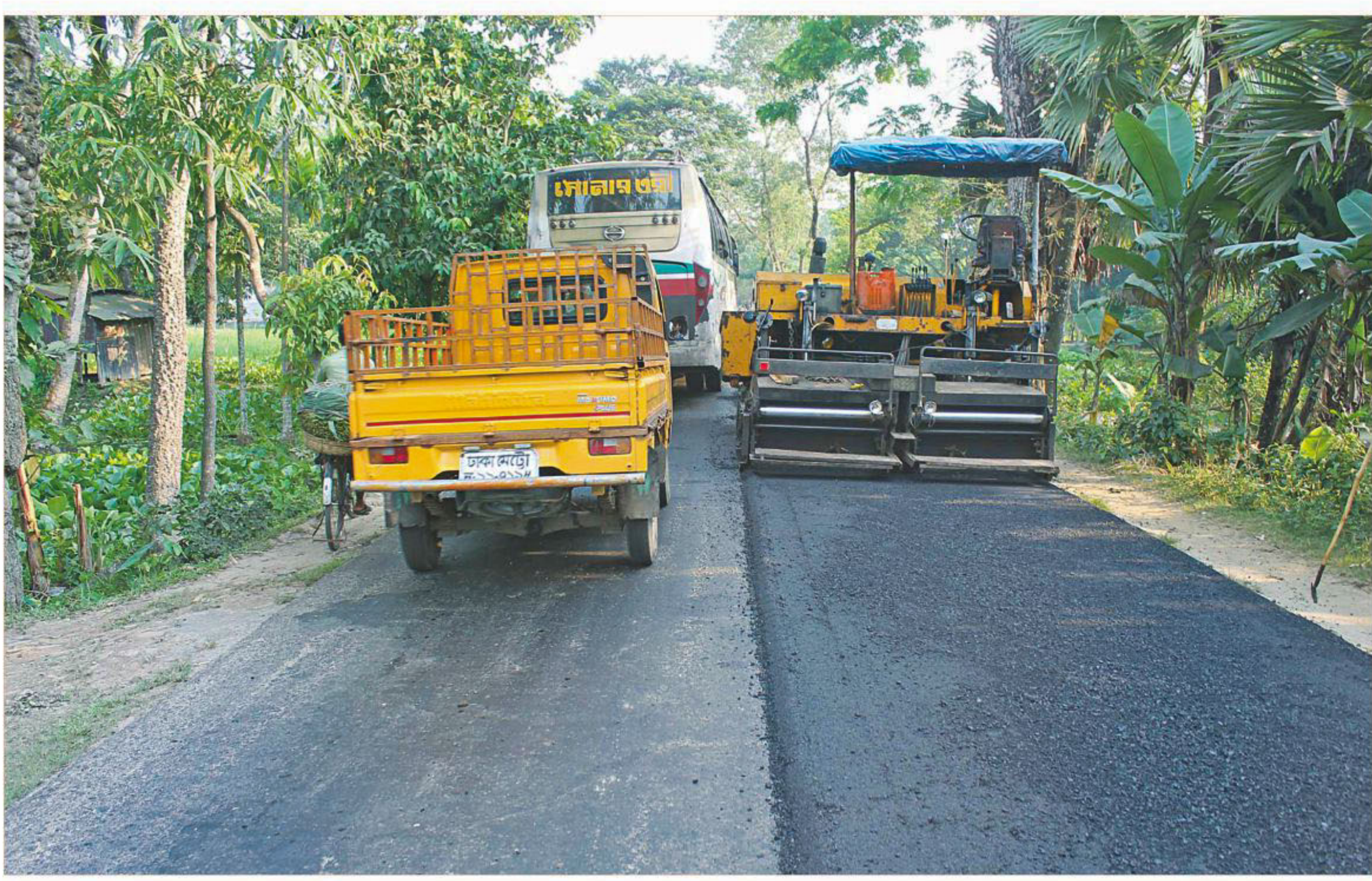
Drivers plying the Barisal-Dhaka highway say vehicles moving on the renovated nine-foot wide lane on the right run the risk of accidents and damage to the lower portion during attempts to overtake others at night. Following the application of a fresh layer of bitumen as part of the ongoing renovation of a 30-kilometre stretch, the renovated surface is some four to 12 inches higher than the strip of ground adjacent to it and four to five inches higher from the untouched lane on the left. The photo was taken at Barisal's Satmile area recently. PHOTO: ARIFUR RAHMAN
