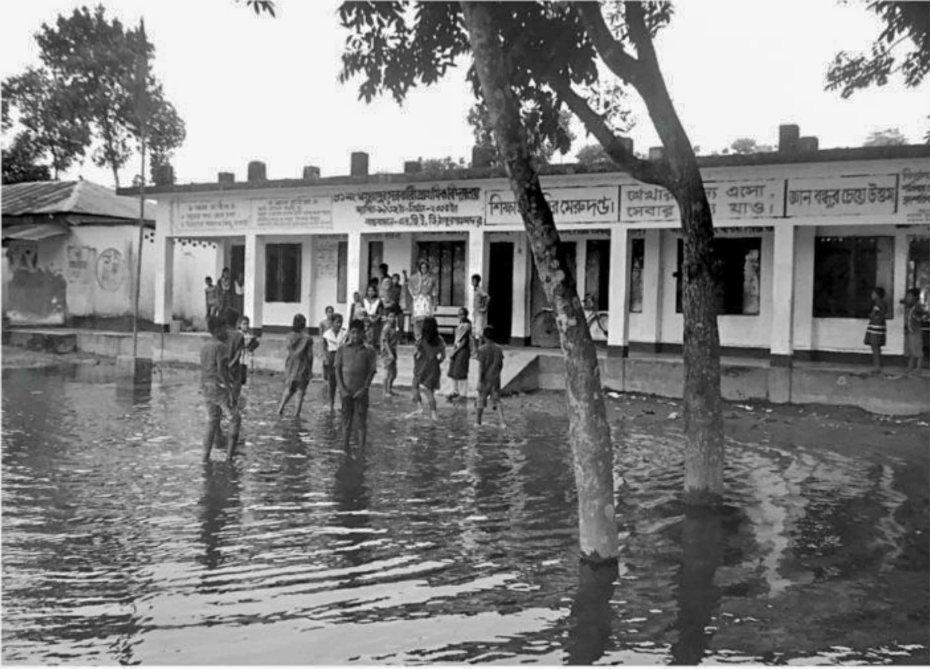
School ground of Mathurapur-1 Government Primary School in Thakurgaon Sadar upazila has remained waterlogged for a couple of months as outlet for rain water got blocked following construction of a road on the eastern side of the ground.
