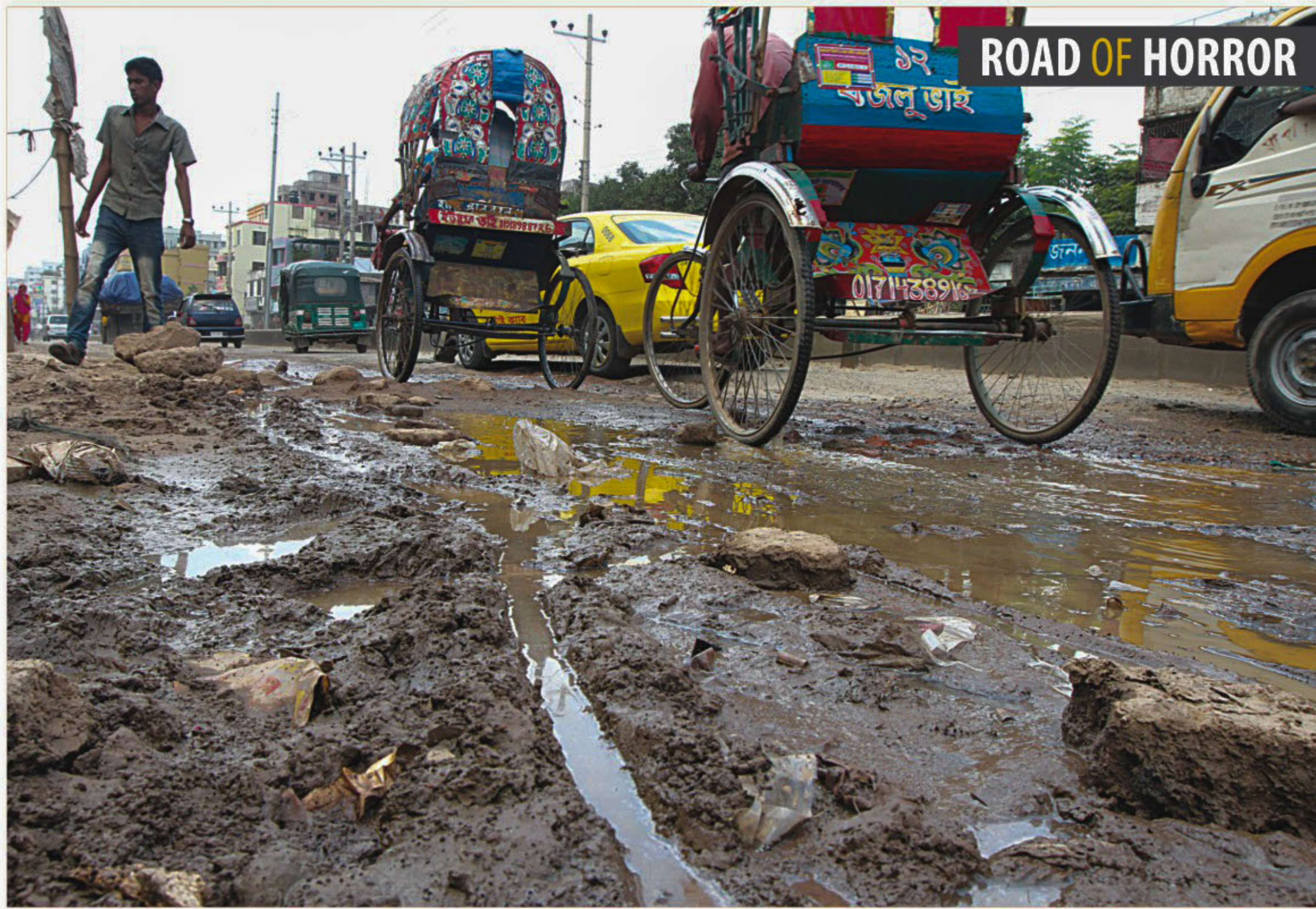
The sorry state of Purabi-Kalshi Road in Mirpur. Hardly any regular maintenance work is done on the road.
