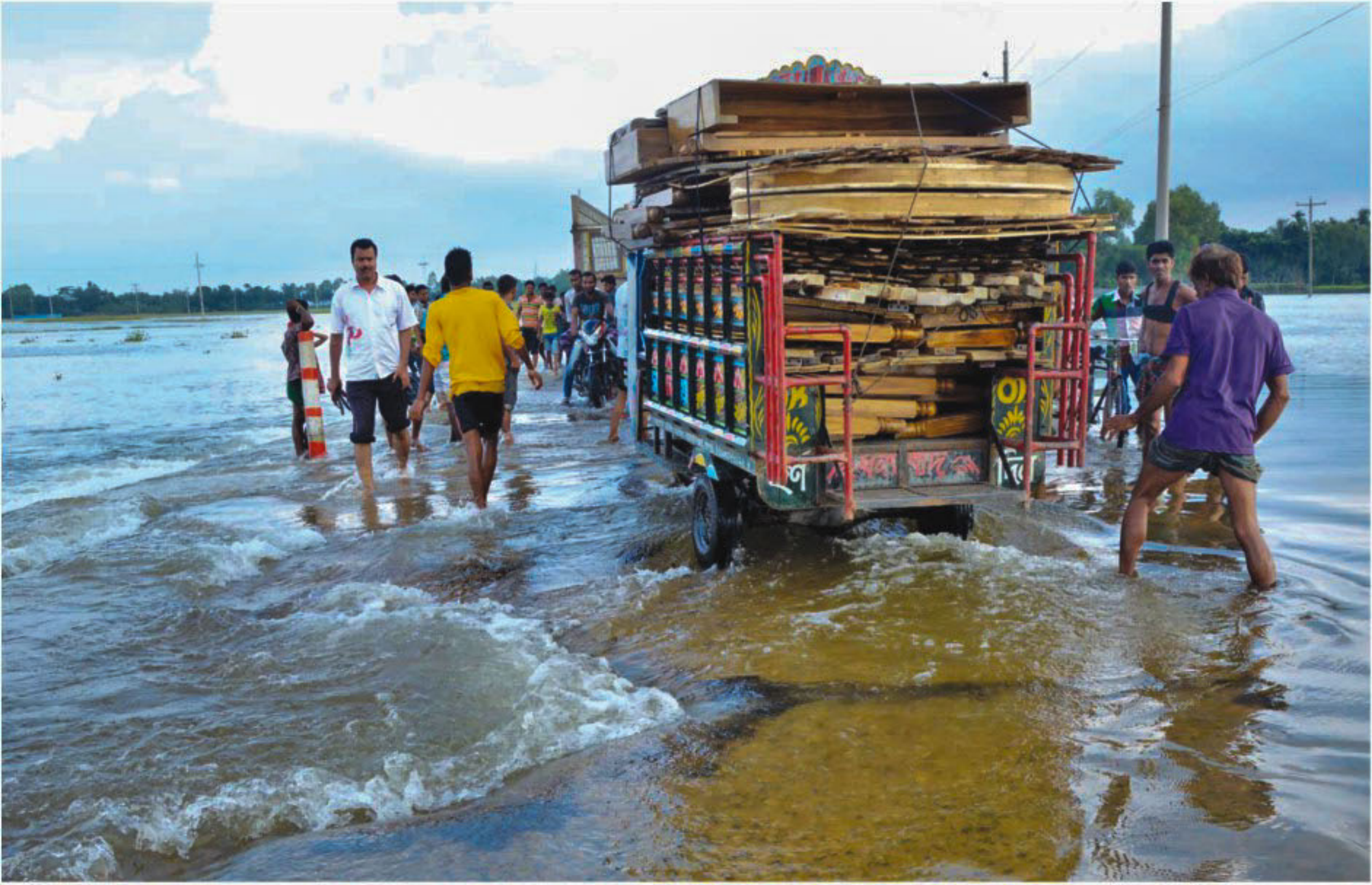
Floodwater inundates Sherpur-Jamalpur Diversion Road at Char Pakkhi yesterday. The movement of heavy vehicles on the submerged road has created potholes making the journeys even more dangerous.
