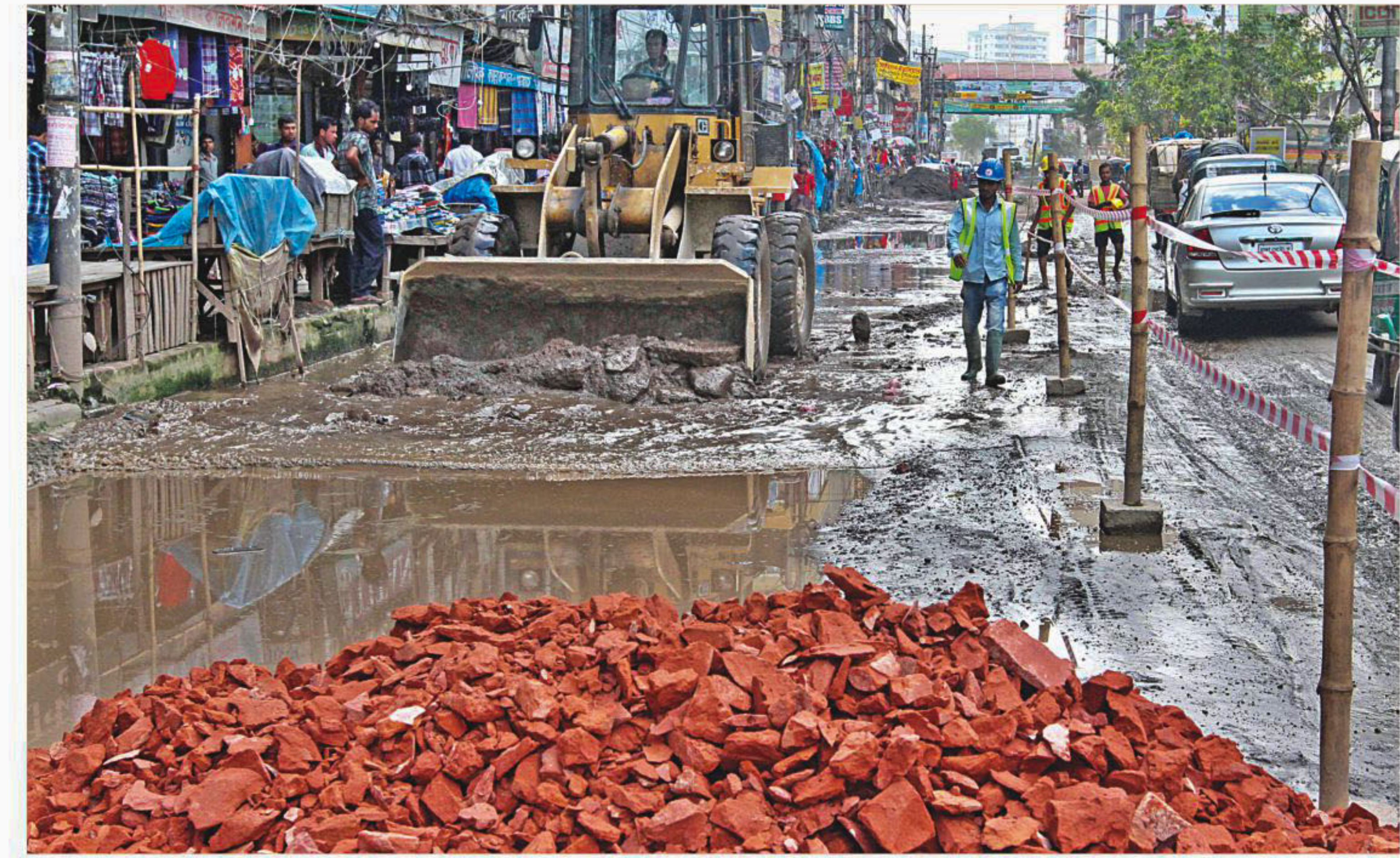
Temporary renovation work underway on the Malibagh-Mouchak road in the capital yesterday, which is battered heavily because of a soil test there several months ago for the construction of Moghbazar flyover. The authorities excavated narrow trenches for the test but did not properly fill those with earth. In the monsoon, the road has turned into a nightmare. The authorities undertook the stopgap measure Thursday night after repeated media coverage of the public sufferings. However, residents of the area are skeptic about how long the road would remain in good shape.
