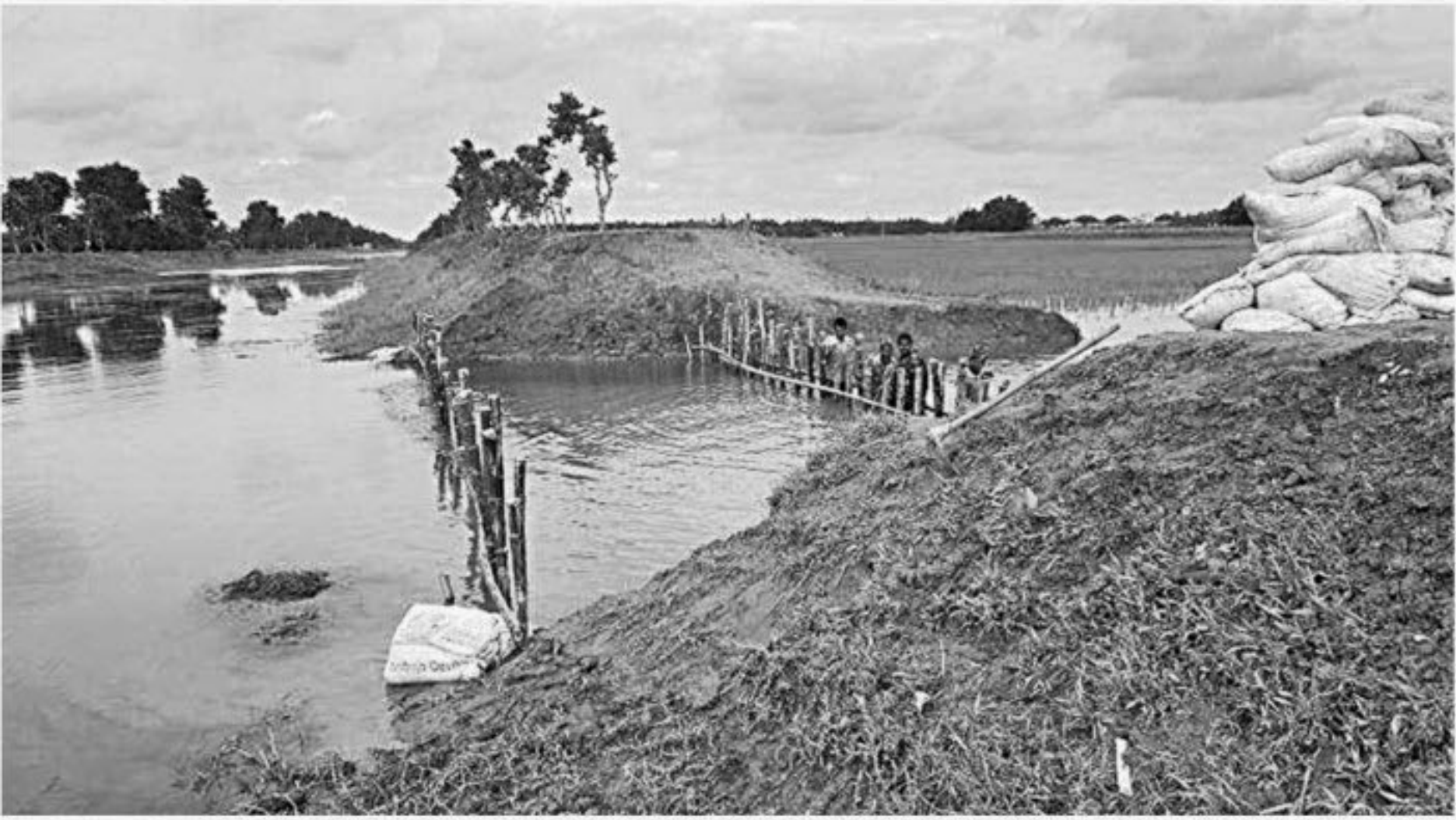
PHOTO: STAR Water Development Board on Thursday started work to repair the breached portion of Nilphamari-Dinajpur branch canal under Teesta Irrigation Project at Dangapara village in Nilphamari Sadar upazila. But aman paddy of around 70 acres of land, flooded due to the onrush of water through the breach, is likely to be fully damaged as the work progresses at a snail's pace.
