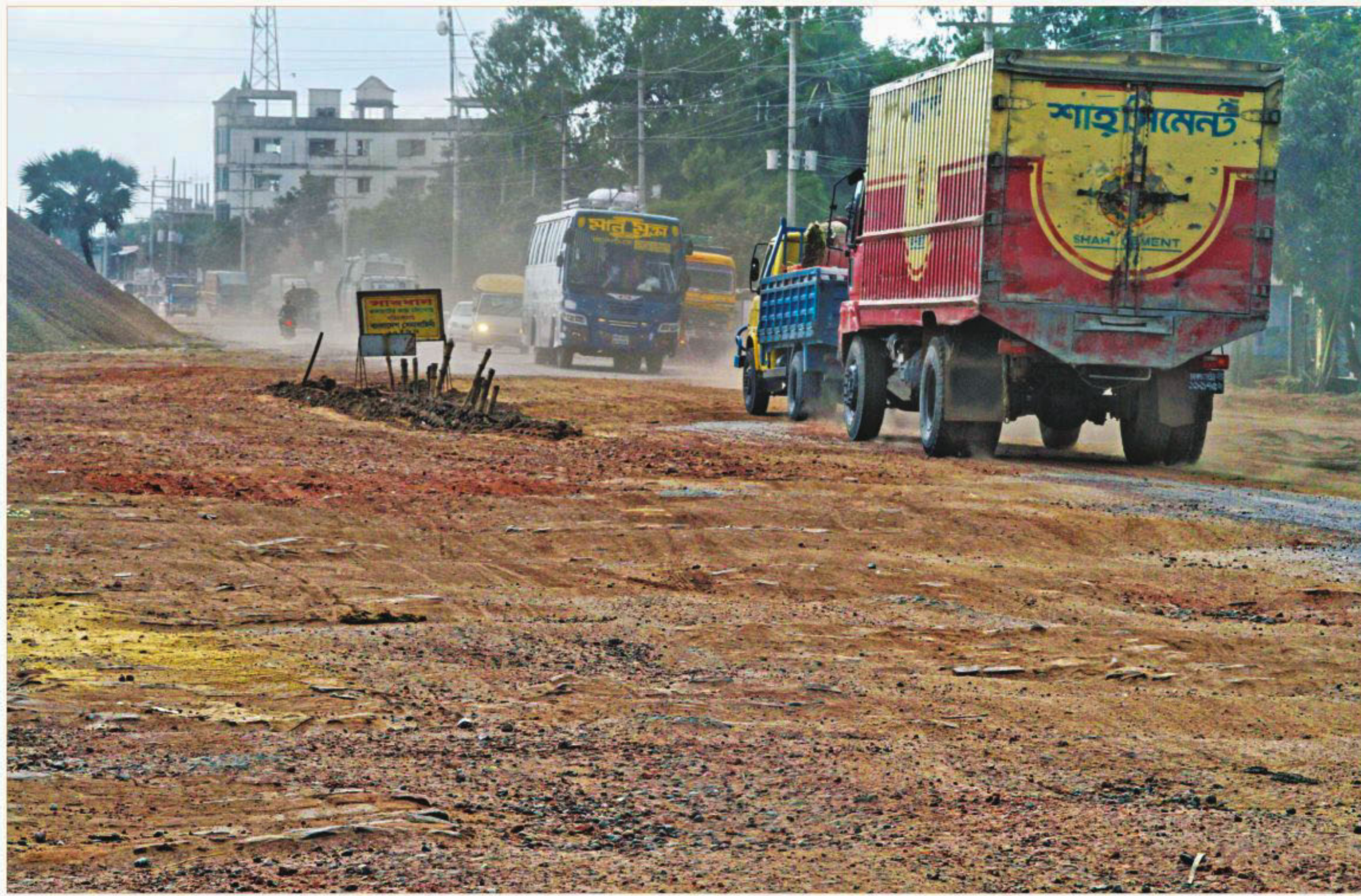
The journey of people during Eid holidays might be as troublesome as it was last year on the Dhaka-Mymensingh route. If the road is not repaired before the vacations, the worn-out surface and potholes at numerous spots will cause a bumpy ride, which means unusually extra travel time and fuel -- not to mention a long tailback. The photo was taken at Masterbari in Gazipur Sadar on Monday. More on page 2. PHOTO: AMRAN HOSSAIN
