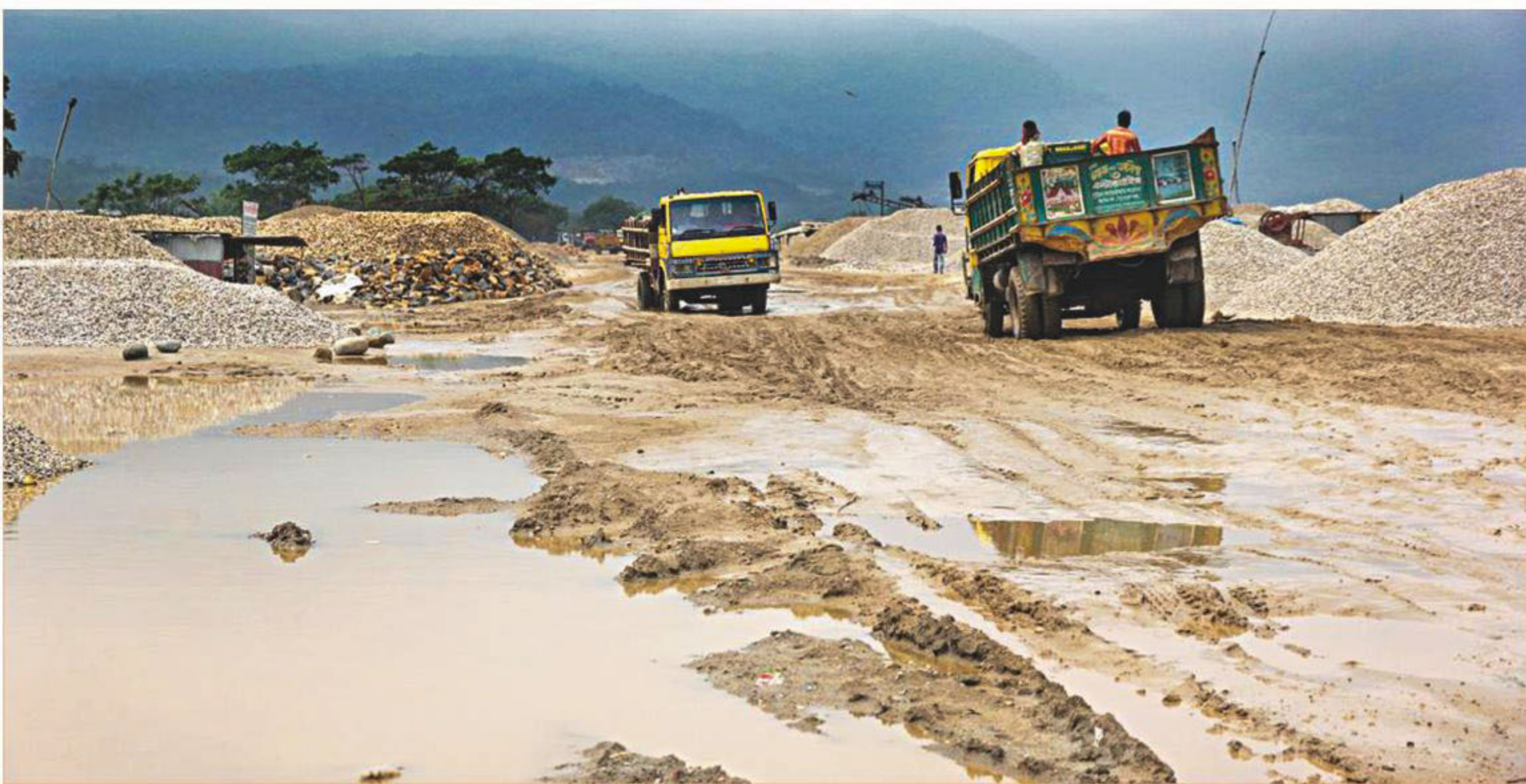
This dilapidated road is actually the major highway that connects Bholaganj, which has the country's biggest stone quarry, with Sylhet city. The 35km road, replete with craters, tremendously disrupts vehicular movement. Roads and Highways Department officials blame plying of overloaded trucks for the battered condition while Sylhet Sadar-Companiganj Unnayan Forum yesterday announced a 17-day programme, including a human chain, from July 11 to pressurise the government for repairing the road immediately. The photo was taken in Bholaganj on Wednesday. PHOTO: STAR
