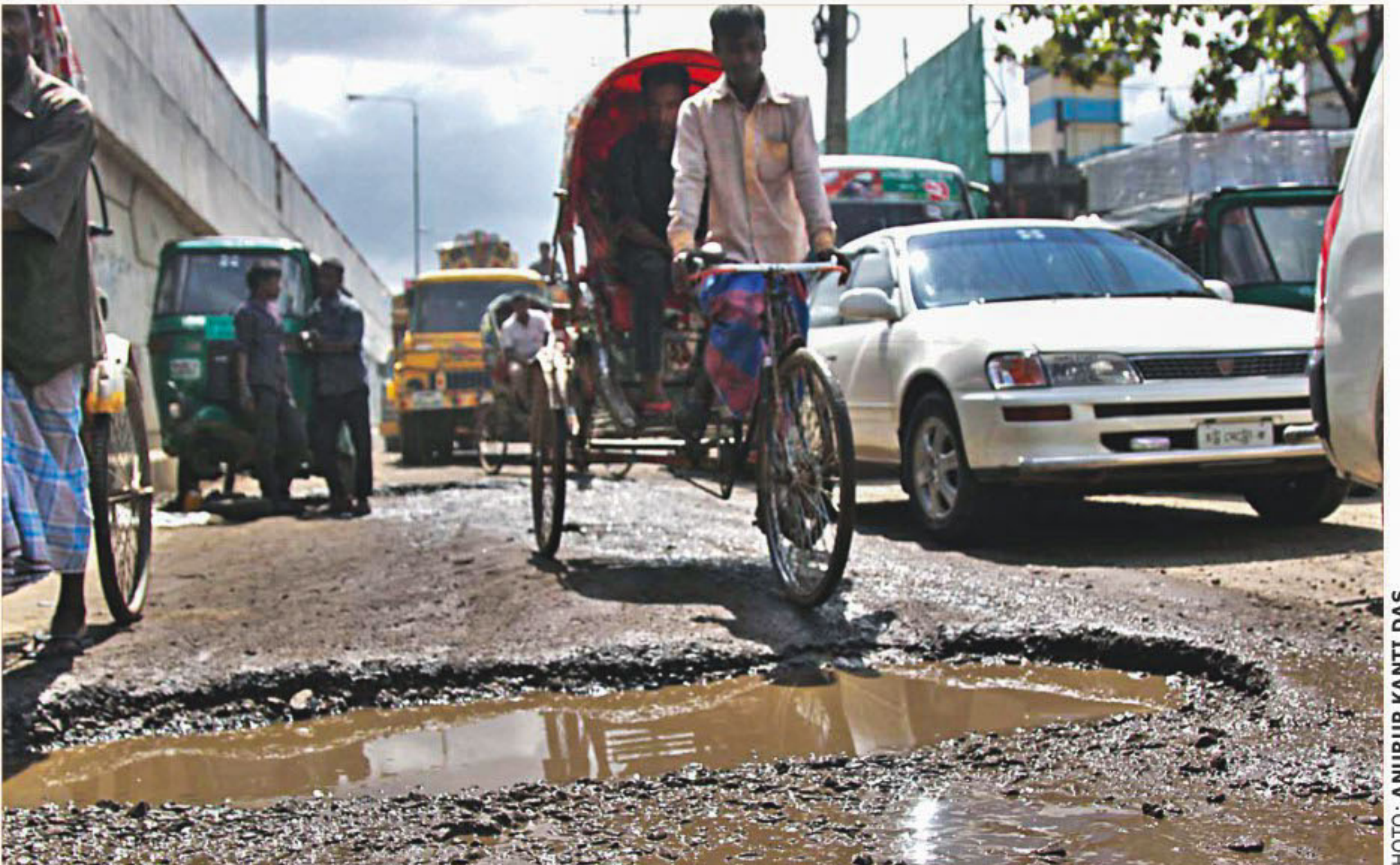
A rickshaw about to hit an inescapable pothole across Arakan Road in Bahaddarhat area, a major thoroughfare in Chittagong city, which has been created due to the use of substandard construction materials during the renovation work done only six months back by the city corporation. This is one cause for traffic jams in the area, as motorists try to avoid the battered part, blocking the passage of the vehicles trailing behind. The photo was taken yesterday.
