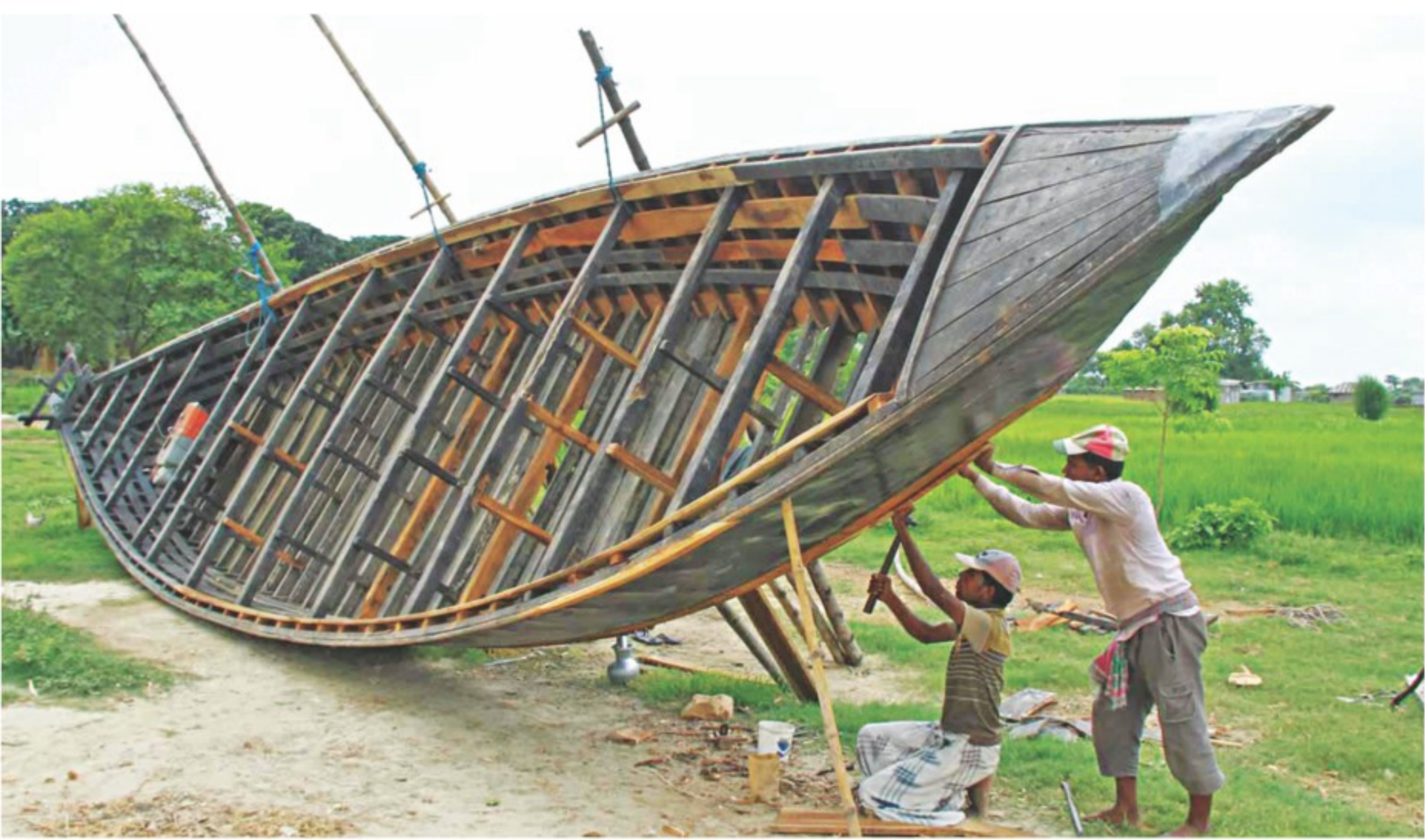
A large country boat undergoing repairs in Charkhanpur of Rajshahi recently. With the beginning of the monsoon, fishermen and the people who make their livelihoods by ferrying goods and passengers across the Padma river have started restoring their vessels to operate those at the time when the river would overflow, deluging vast tracts of land and suspending road communication. Last year, these people witnessed severe flooding with water submerging even parts of Rajshahi city, but many who did not own boats or have their boats ready could not seize on the opportunity of making some extra bucks during that period.
