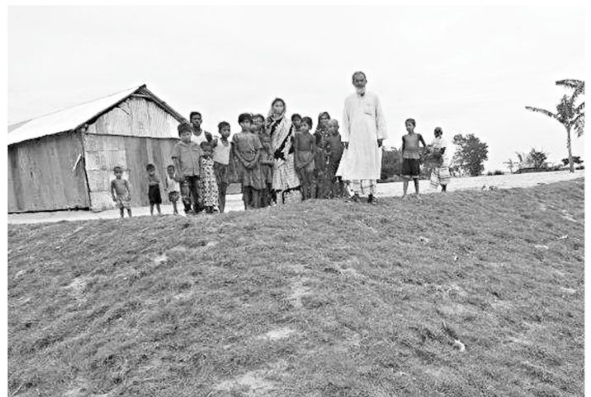
A newly constructed earthen 'killa', a safe place higher than usual floodwater level, at Kisamoter Char in Teesta River basin area in Dimla upazila of Nilphamari. UNDP provided financial, technical and monitoring support for construction of the shelter for people of the area in times of flood.
