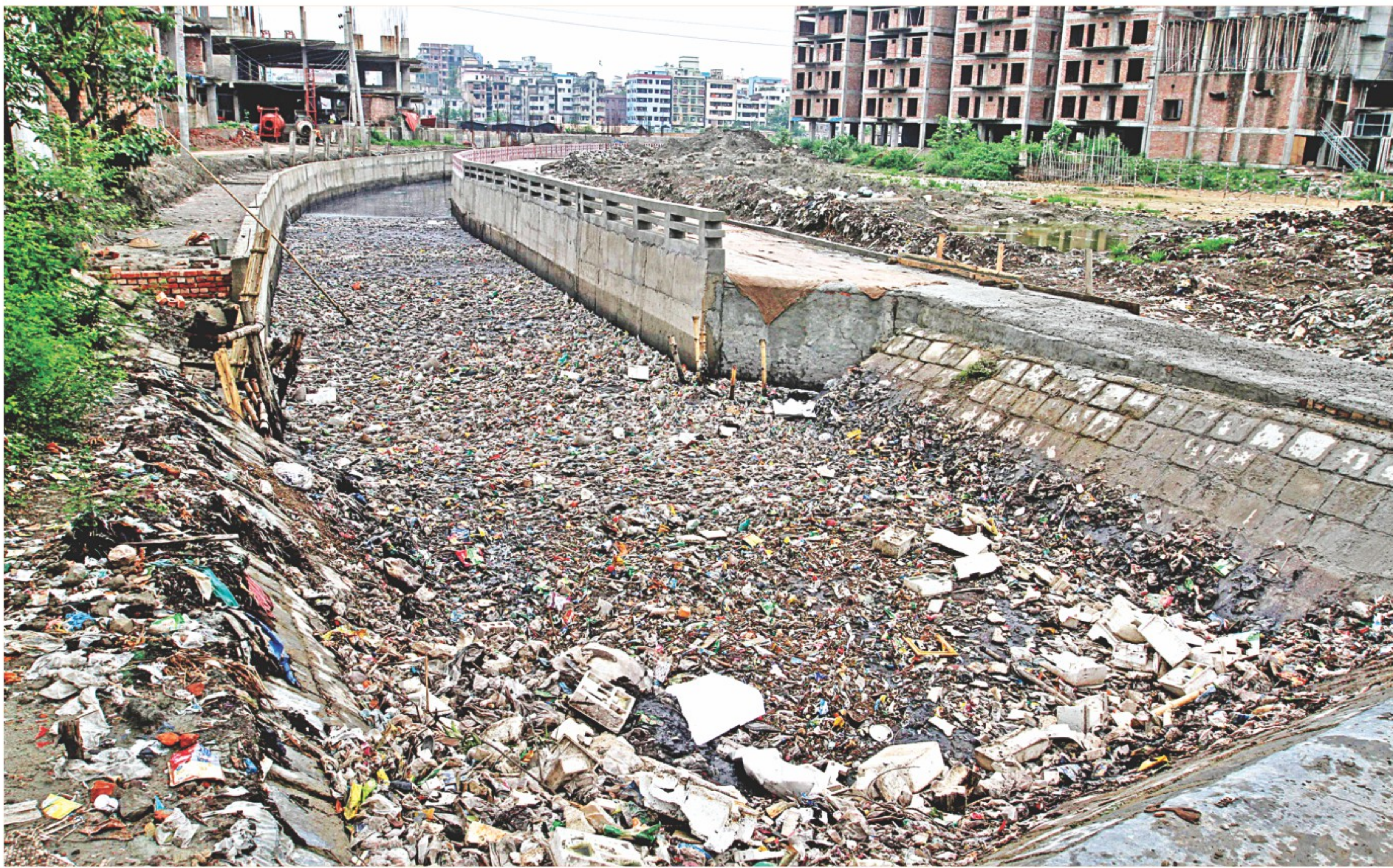
Rubbish has clogged the newly constructed drainage canal in the capital's Hazaribagh. Though it has started to rain, most of such outlets in Dhaka city remain choked with garbage or dried sludge, making stormwater drainage immensely difficult and consequently causing waterlogging. The photo was taken recently.
