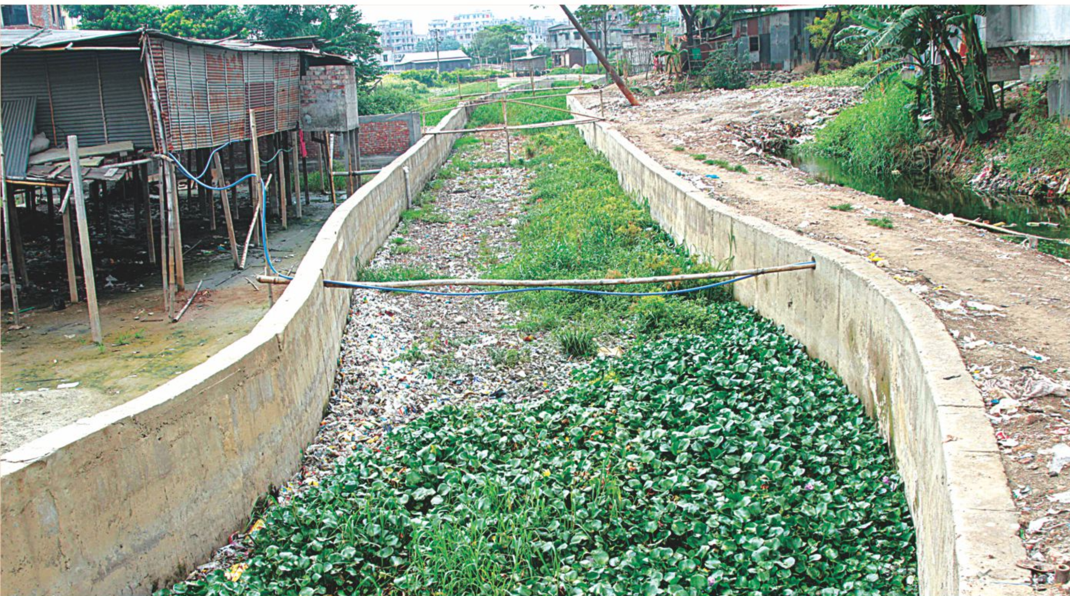
Dried sludge and household discards thickly deposited in this stormwater drain of Wasa in the capital's Madinabagh is lush with water hyacinths and grass. If its original depth is not restored before the upcoming monsoon due in just two weeks, a vast area encompassing the neighbourhoods of Bashabo, Ahmedbagh, Rajarbagh, and Sabujbagh is surely to see severe waterlogging, bringing tremendous sufferings to the residents, as it is the only major rainwater outlet there.
