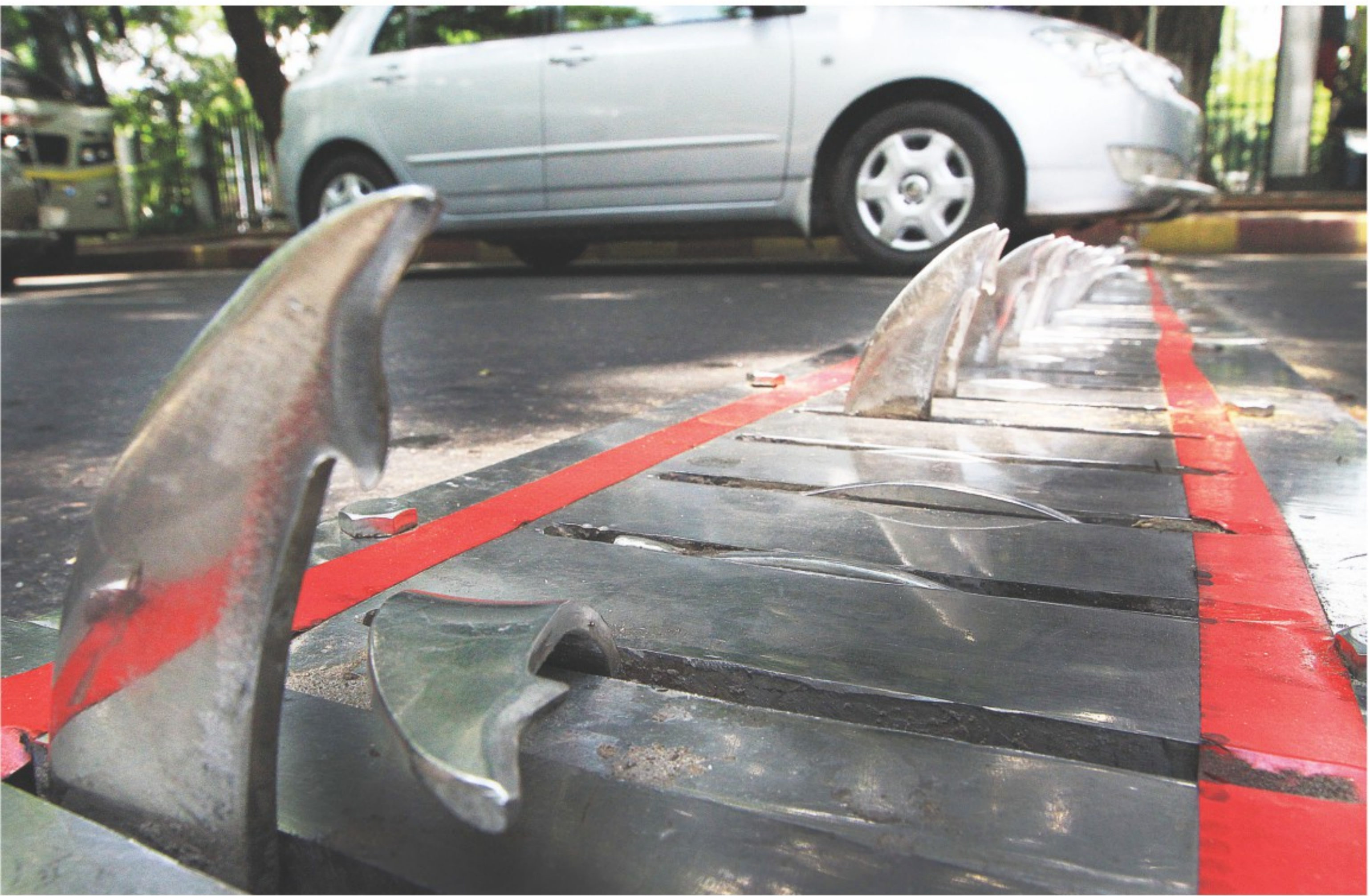
Spikes of this retractable spike strip were already broken yesterday just two days after it was installed with a lot of hoopla on Hare Road in the capital to prevent motorists from driving on the wrong side of the road. PHOTO: PALASH KHAN
