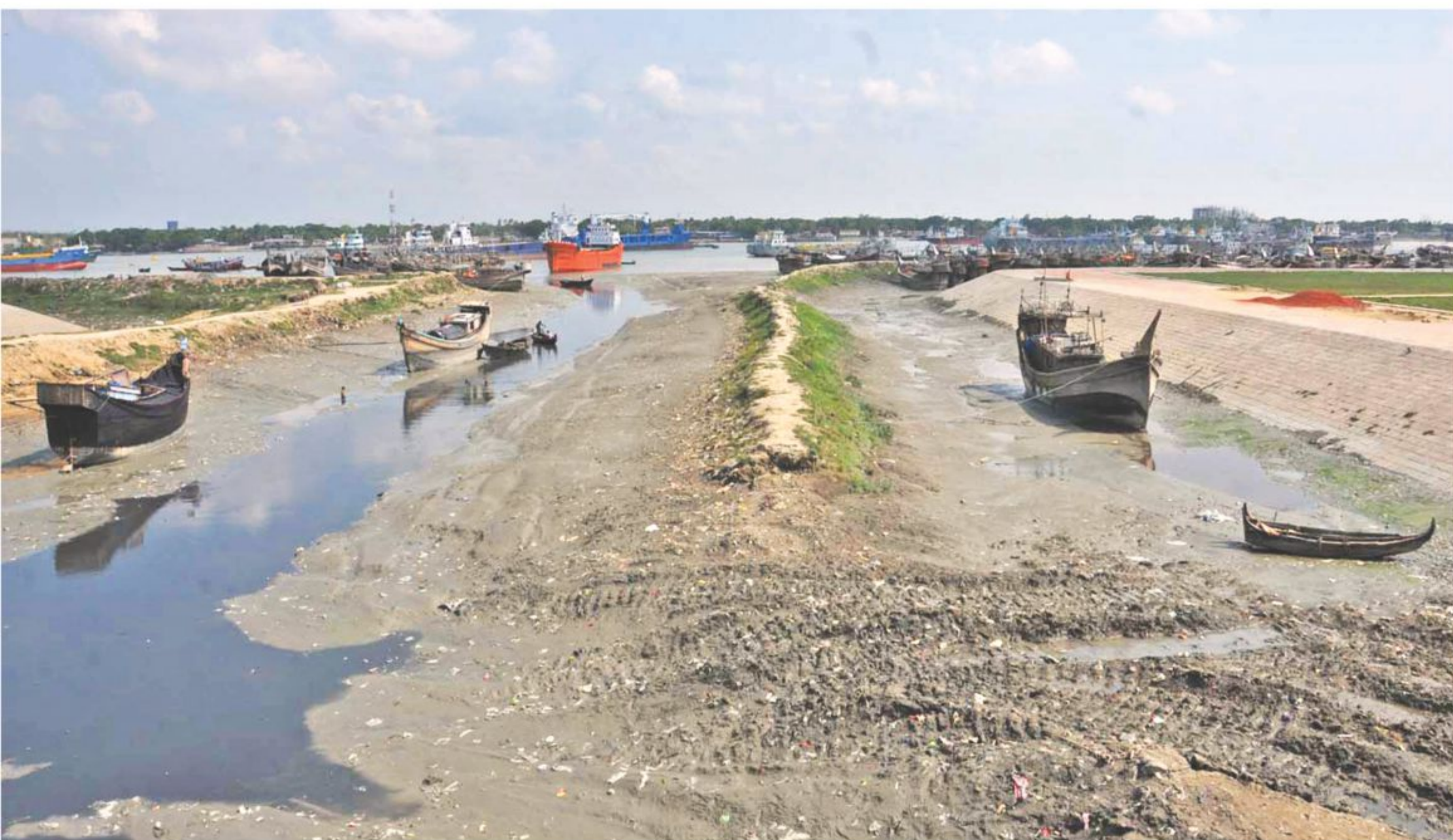
The Chaktai canal, which flows into the river Karnaphuli, is a major water body as it ensures storm water drainage of Chittagong city. But silts extracted after the Karnaphuli dredging have clogged the canal. During low tide, it almost loses navigability, suspending movements of boats.
