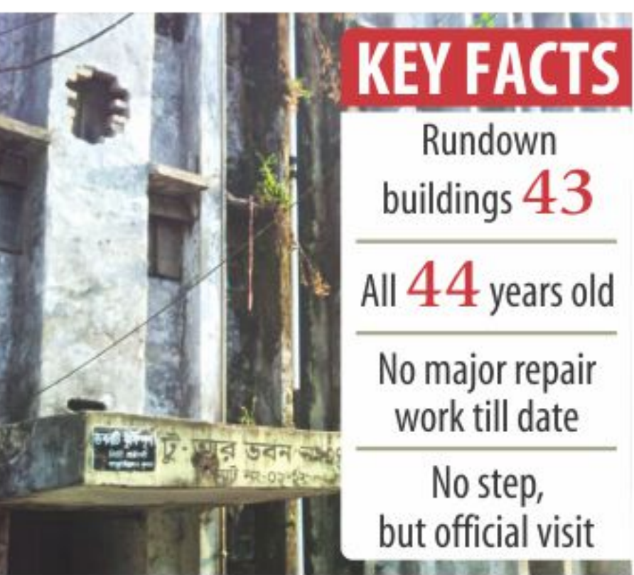
Part of a risky building.
