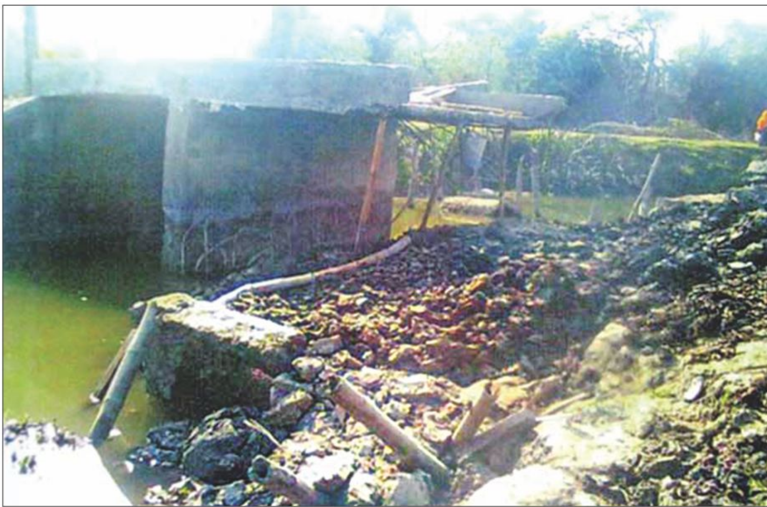
The rubble left after a portion of a culvert collapsed at Hosnabad of Dashmina upazila in Patuakhali. Locals claimed that the culvert collapsed just a month after its construction because the contractor used sub-standard materials. PHOTO: STAR
