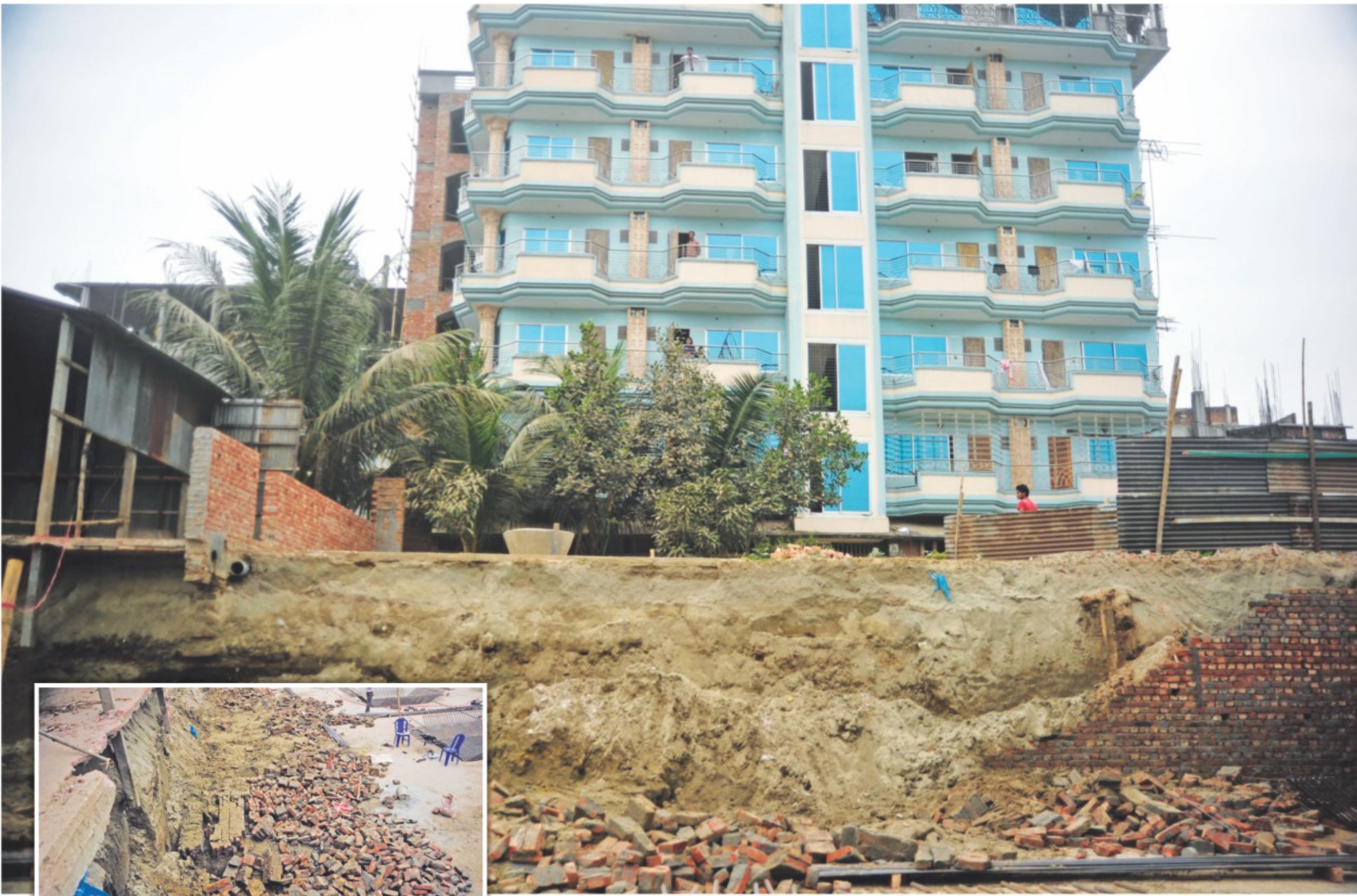
The collapse of this brick wall in Badda in the capital yesterday claimed the lives of two construction workers and sent two others to hospital. Instead of using pilings to stop dirt sliding into the trench for the foundation, the brick wall was built, inset.
