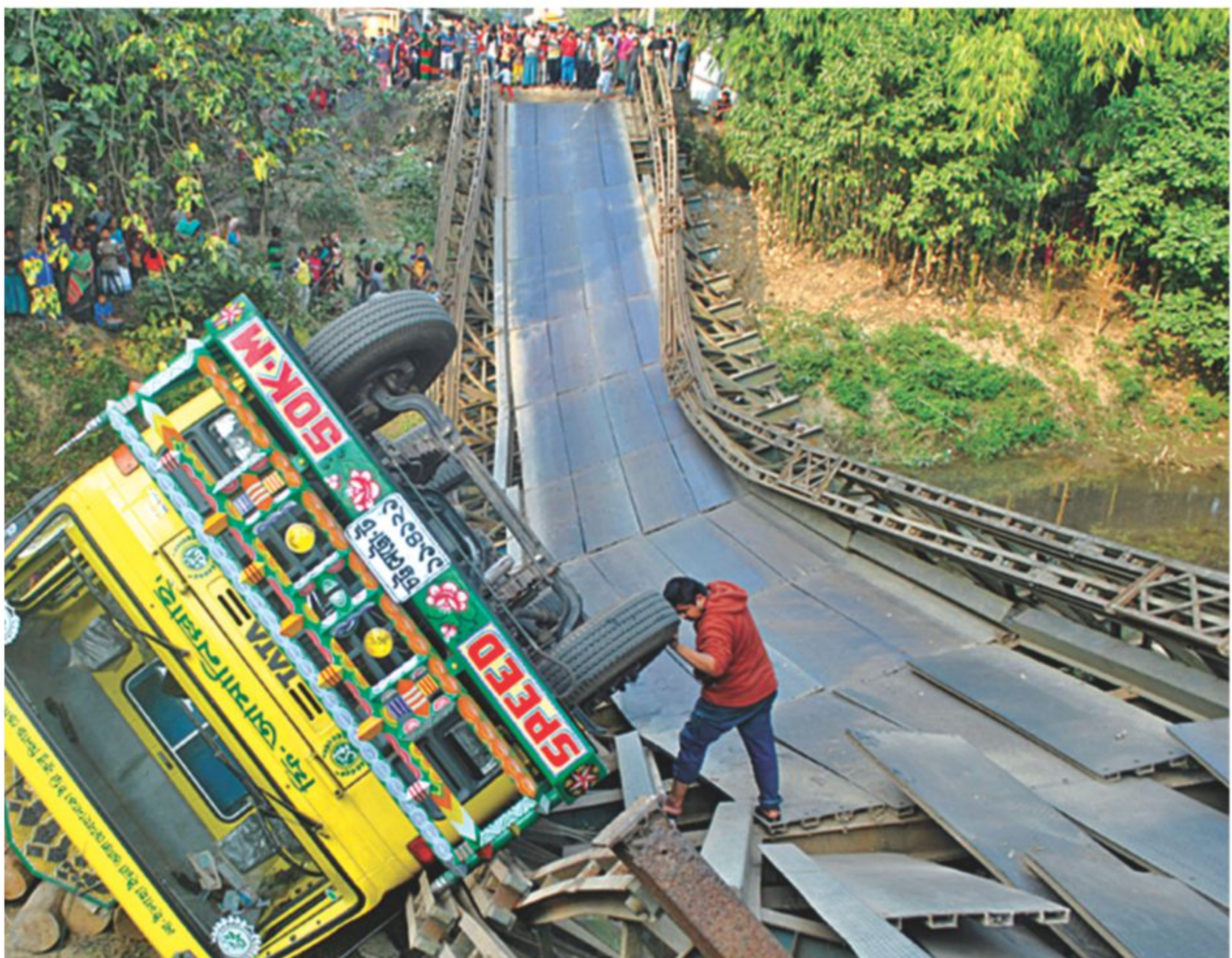
PHOTO: STAR This bailey bridge at Khagrapur in Khagrachhari Sadar upazila collapsed under the pressure of a timber-laden truck on Tuesday afternoon, snapping road communication with Dighinala upazila of Khagrachhari and Baghaichhari and Longudu upazilas of Rangamati district. Despite dilapidated condition of the bridge for several years, authorities concerned had conducted only minor repair works, locals said.
