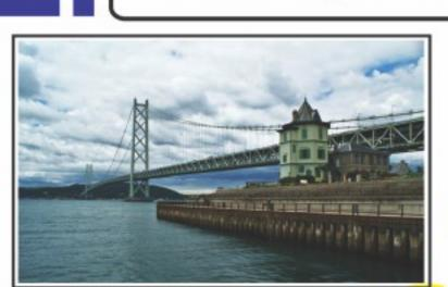
Akashi Strait Bridge in Japan has the longest central span, 1991 metres. It connects two islands of Japan. Its total width is 30 metres and length is 3991 metres which is the highest for any suspension bridge. The total cost of the bridge was 4.3 billion dollars. In terms of supporting towers which rise upto 282.2 metres, it is also the tallest bridge. It took two million workers ten years to complete the bridge.
