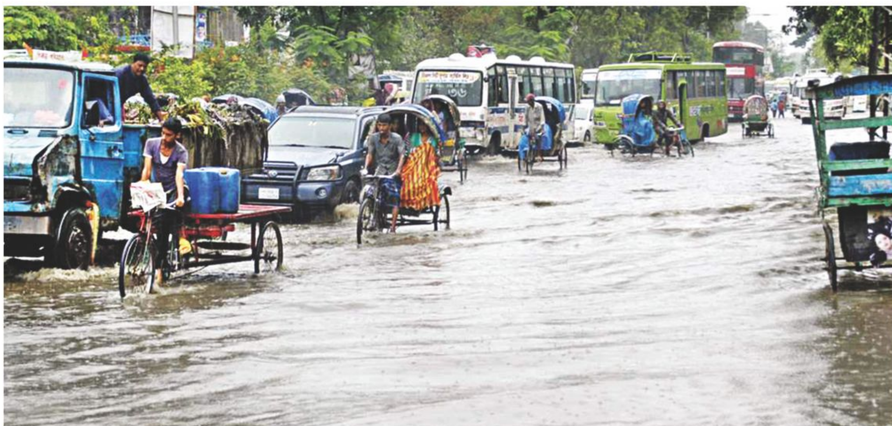
Even light rains cause flooding of the road in the capital's Mirpur-12, which lacks a proper drainage system. The photo was taken yesterday.
