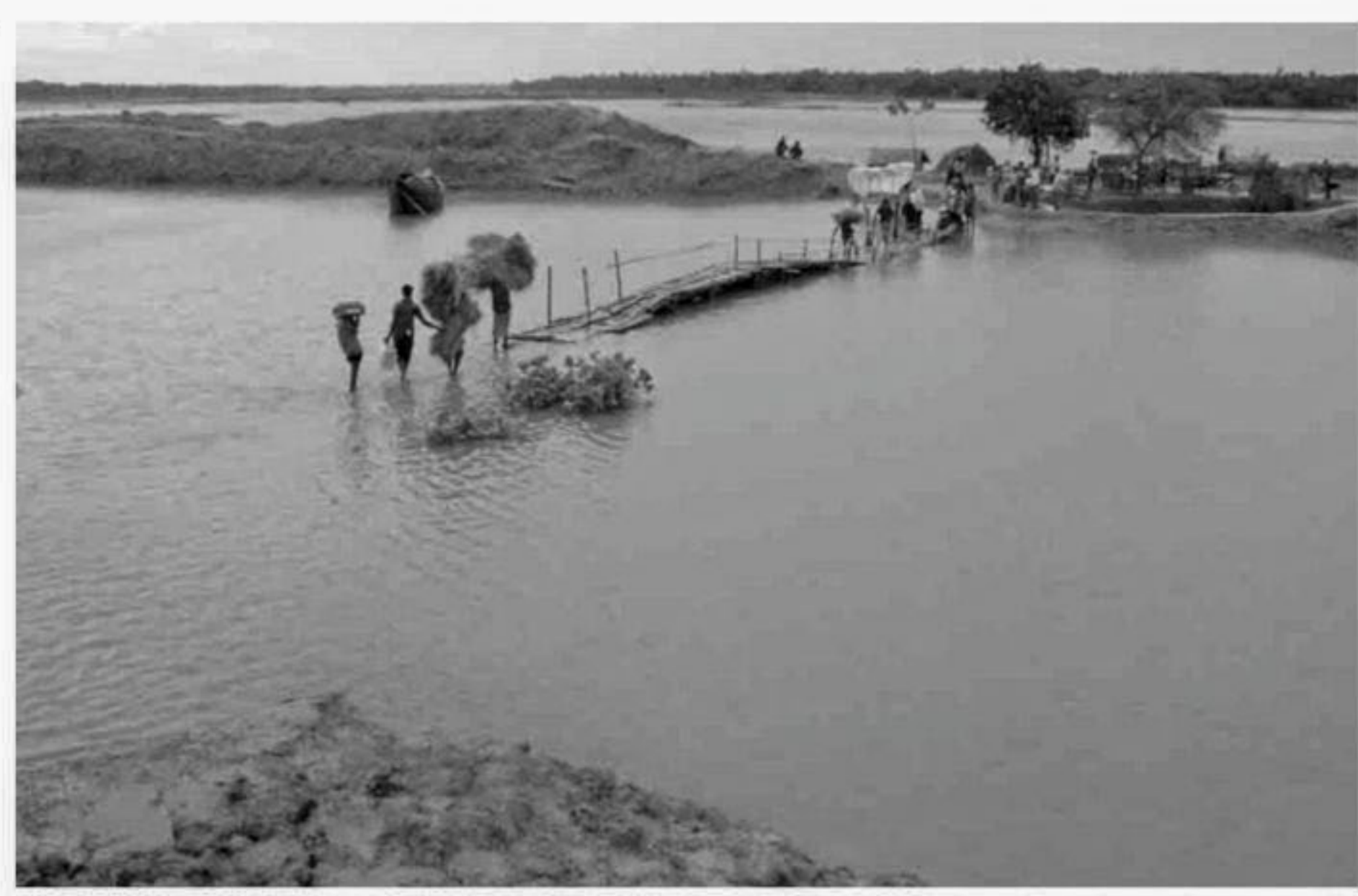
PHOTO: STAR Locals, including school kids, cross Shalikhra River in Tala upazila under Satkhira district using this risky bamboo structure in the absence of a permanent bridge there.
