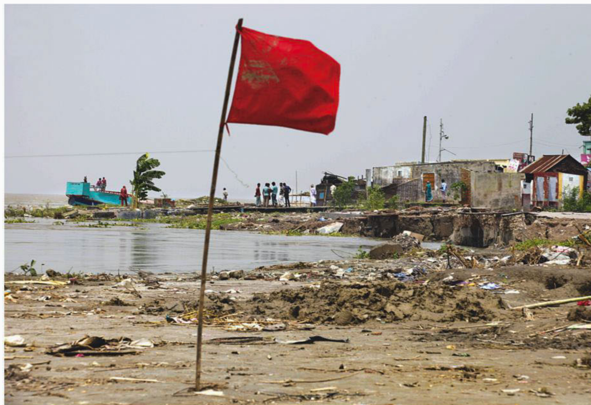
A red flag warning people that the area is at risk to river bank erosion at Mawa ferry terminal as the mighty Padma continues to devour the terminal area, top right, and people evacuate the area dismantling their homes, bottom right. The photos were taken on Wednesday.
