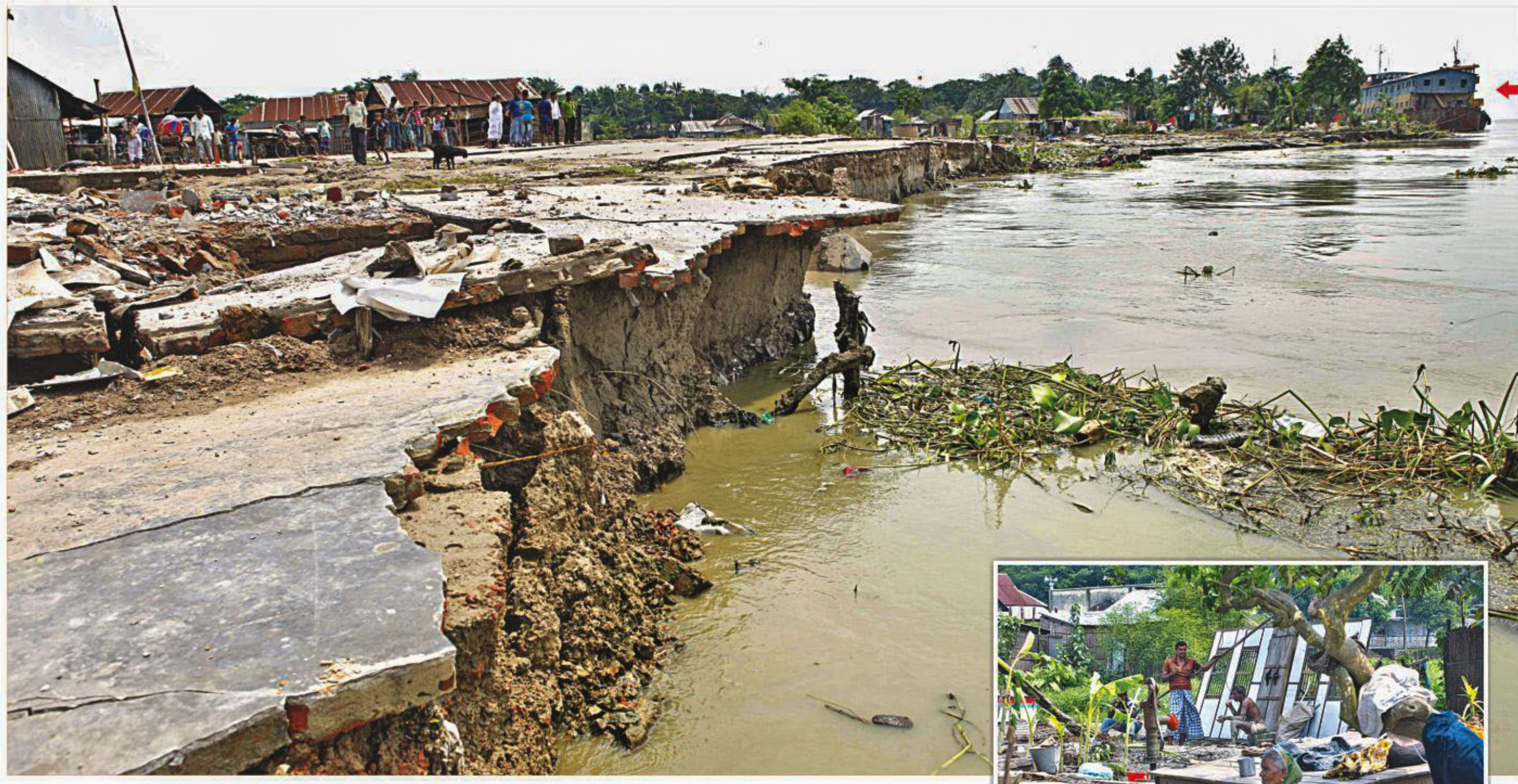
The mighty Padma devours land at Mawa ferry terminal very close to a pontoon seen in the top right corner of the photo while people dismantle their homes, inset, and move elsewhere. The photos were taken on Wednesday.
