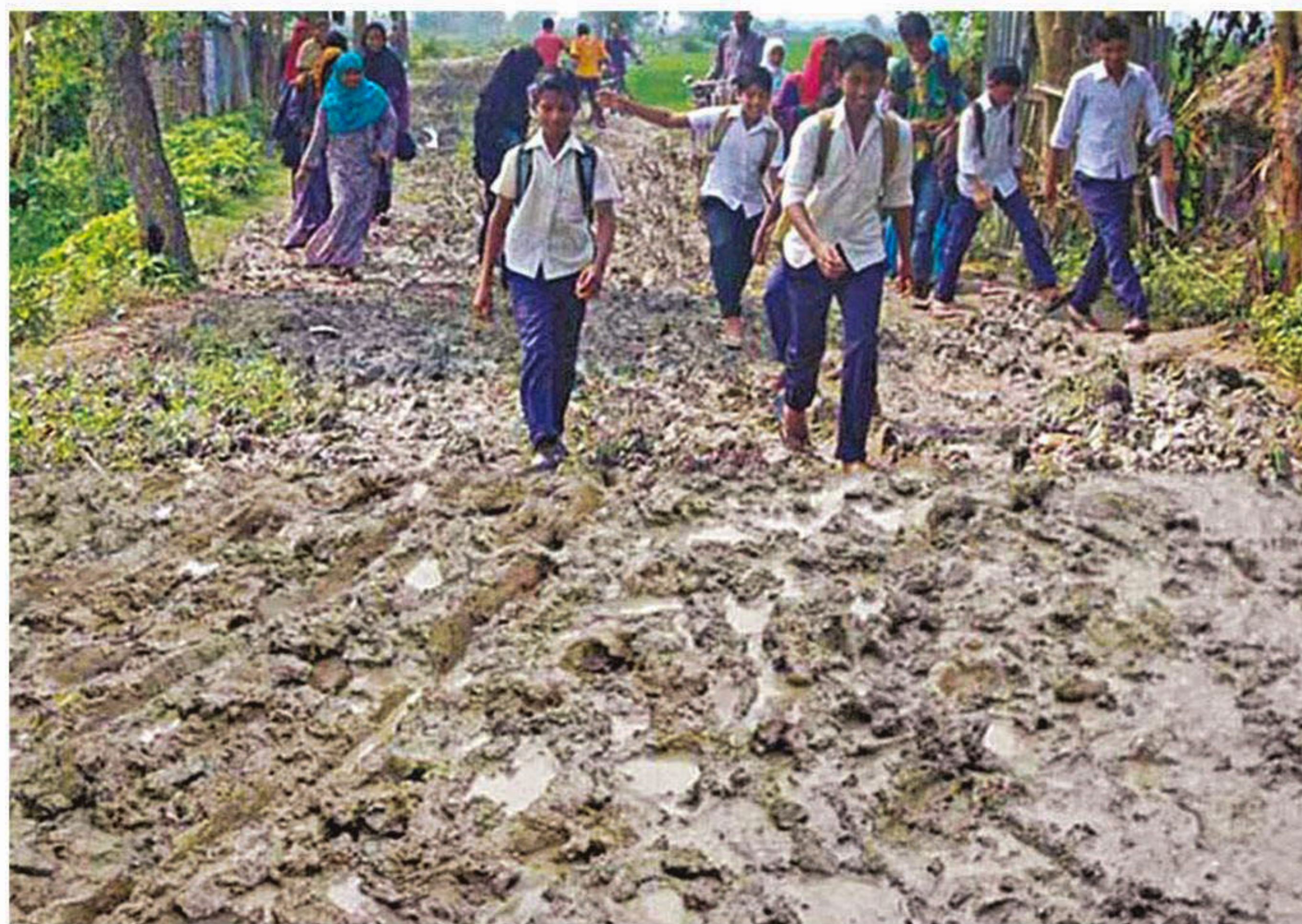
The appalling state of a road at Singa of Harinakundu municipality in Jhenidah. The muddy stretch of about 750 metres forces many villagers to take a detour of 14km to get to Harinakundu.
