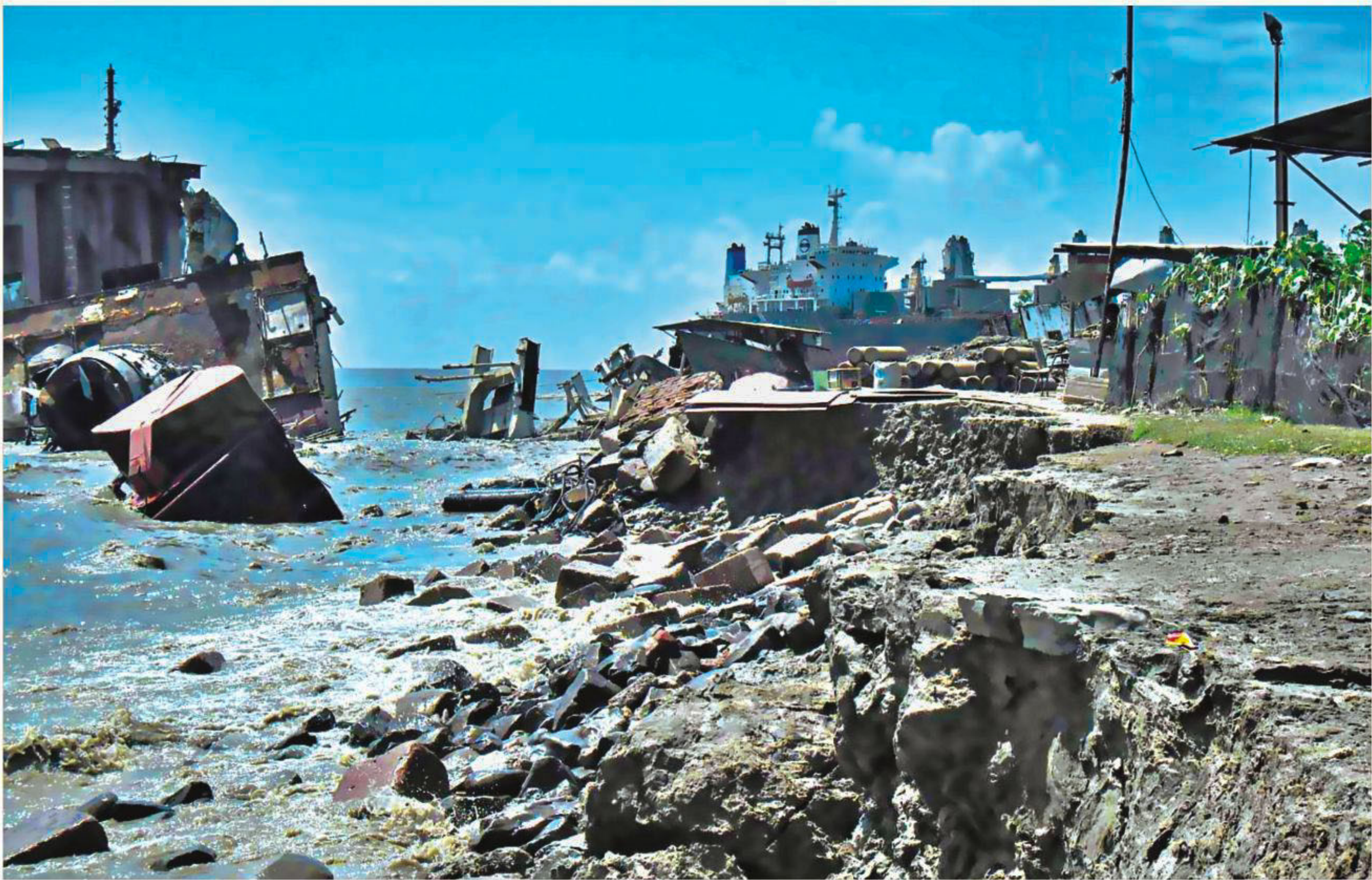
The Sitakunda embankment in Chittagong lies badly damaged by ship-breaking activities, mostly movement and dumping of heavy metal parts from scrap ships. Wide gaps have developed on the dyke and through them seawater rushes into adjoining Joramtol area at high tide. The photo was taken a few days ago.
