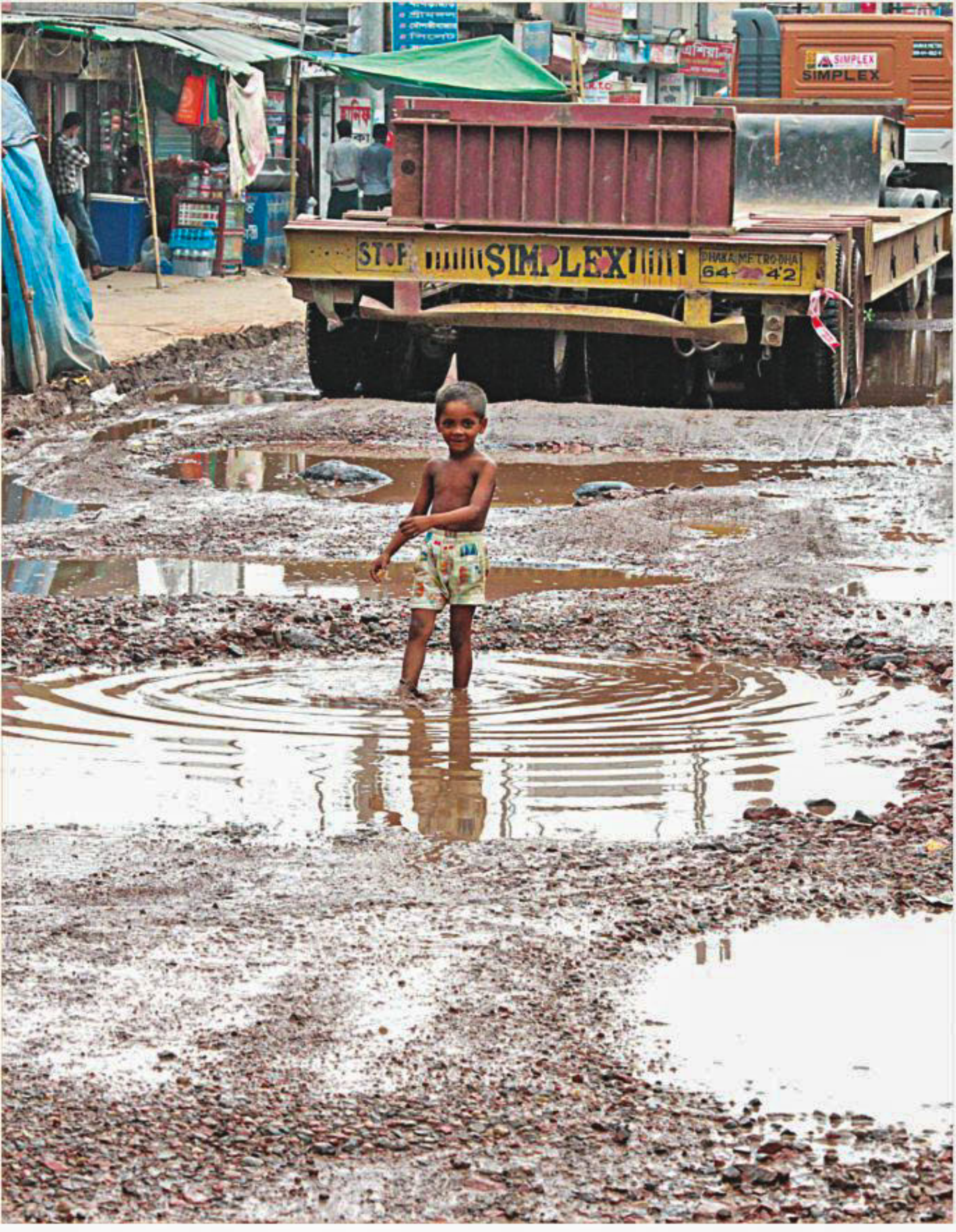
Muddy water collects on craters, created following the movement of heavy vehicles working on the construction of a flyover, on this road near RK Chowdhury University College in the capital's Sayedabad. The photo was taken yesterday. PHOTO: SK ENAMUL HAQ
