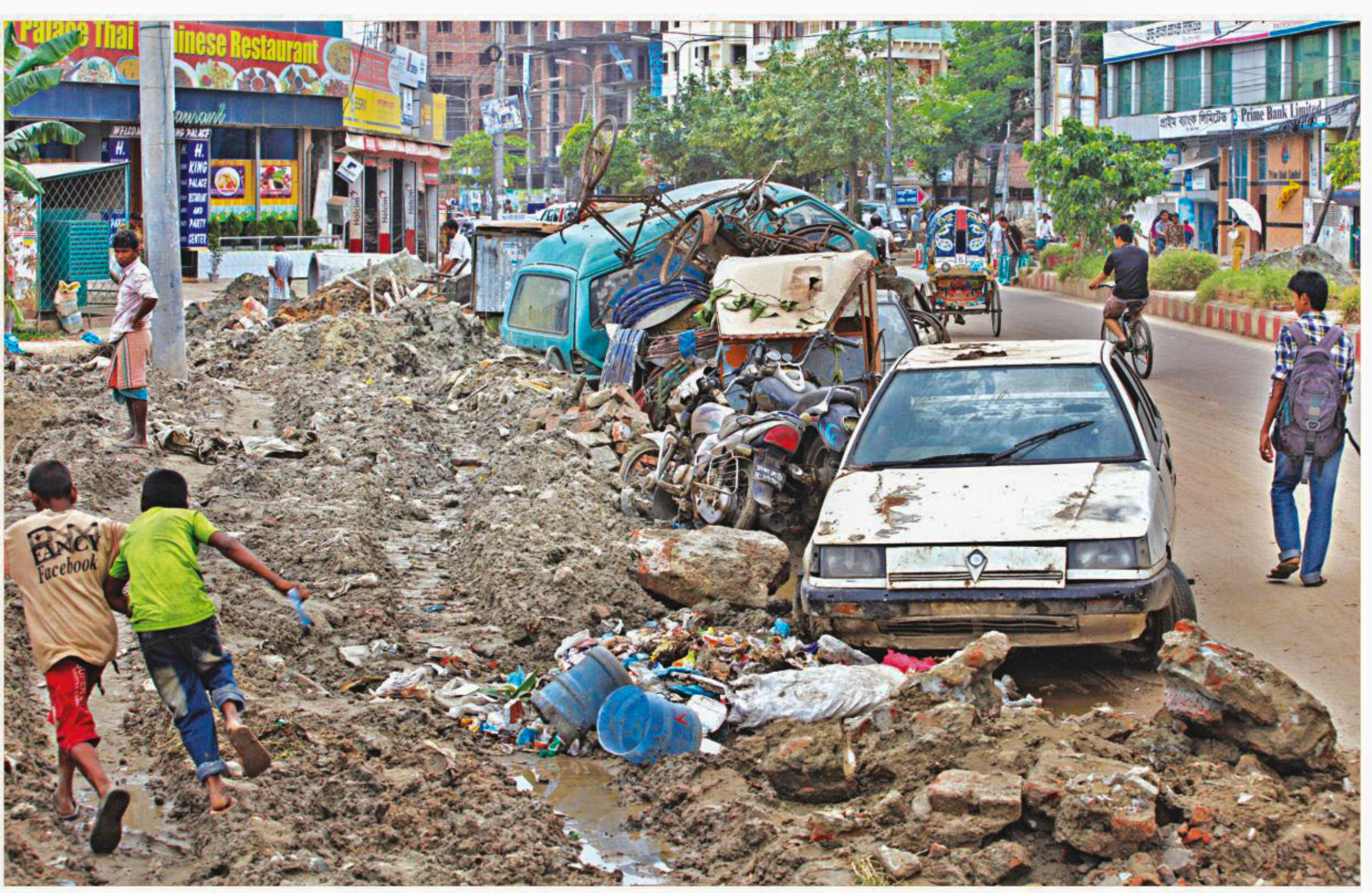
A sizable portion of the Shyamoli-Mohammadpur road opposite Adabar Police Station has long been occupied by seized vehicles dumped by Adabar police, earth dug for building a sewer by Dhaka North City Corporation, and garbage thrown by locals. This is causing hindrance to the movement of vehicles, thereby suffering to the commuters. The photo was taken yesterday.
